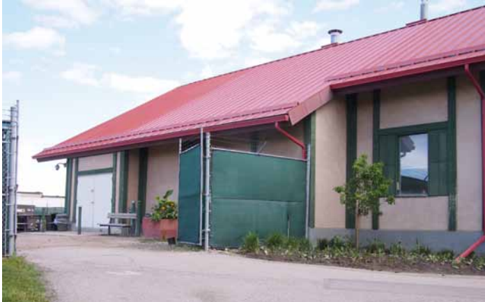
Maintenance yard south entry
