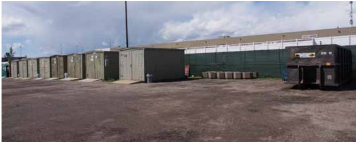
Maintenance yard enclosure
