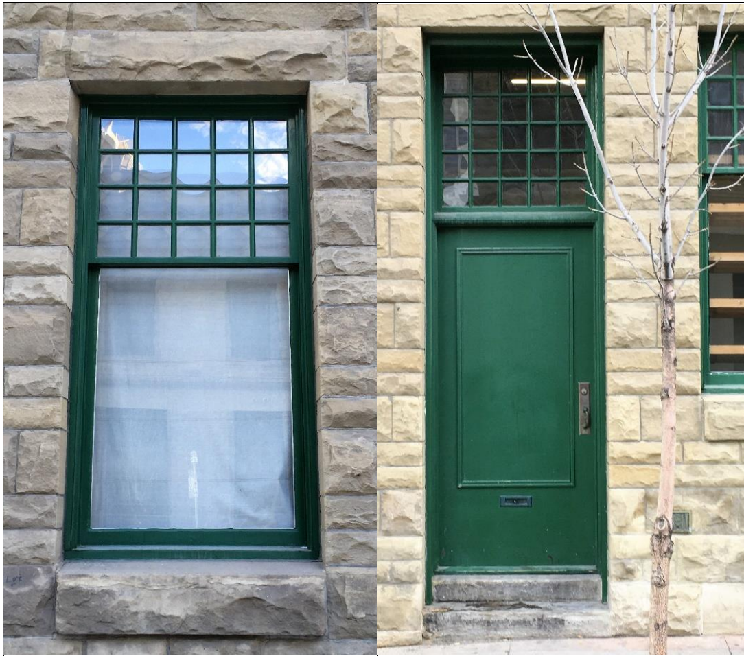
Image 1.9: Typical fenestration, sandstone lintel and sill.
