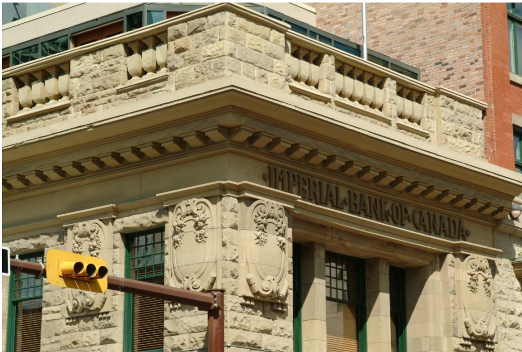
(Image 1.6: Detail of parapet, pressed-metal cornice and frieze)
