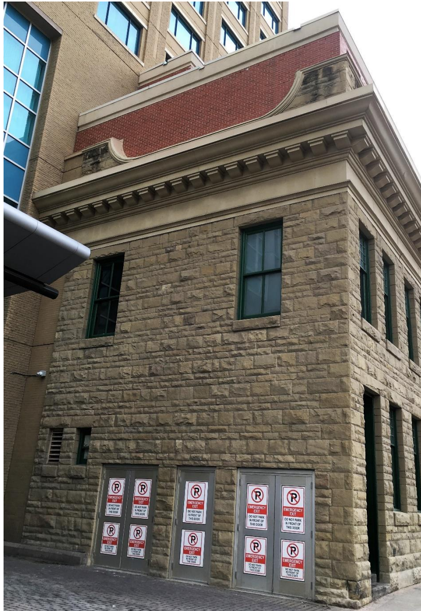
(Image 2.1: North façade, sandstone exterior; 'U'-shaped parapet, pressed-metal block-modillion cornice and frieze)
