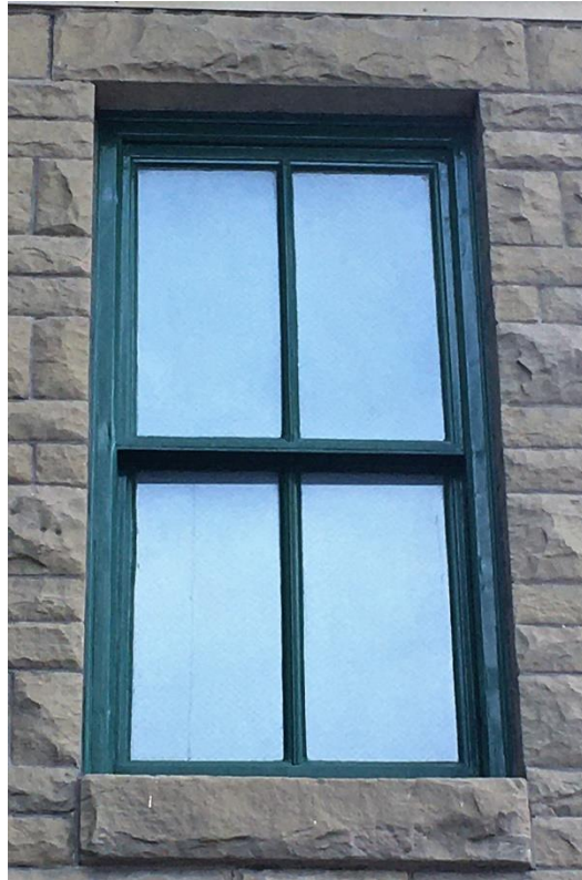
(Image 2.2: Typical upper storey fenestration, sandstone lintel and sill)
