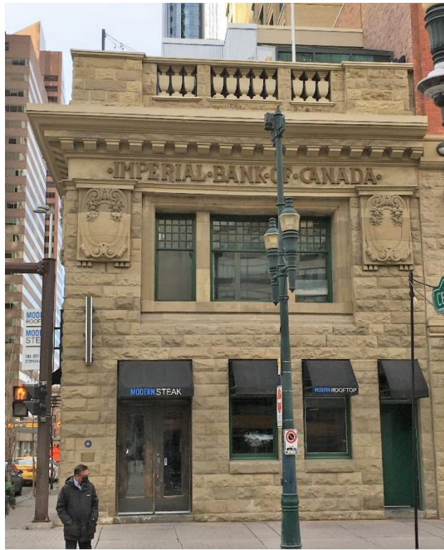
(Image 1.3: South façade)
