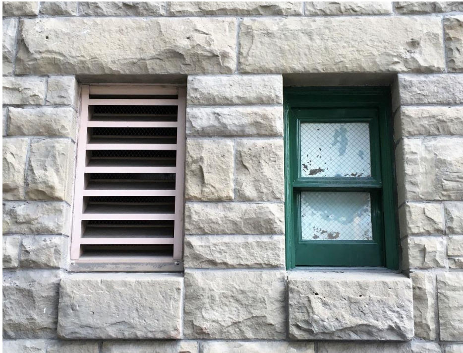
(Image 2.3: Lower storey fenestration, sandstone lintels and sills)
