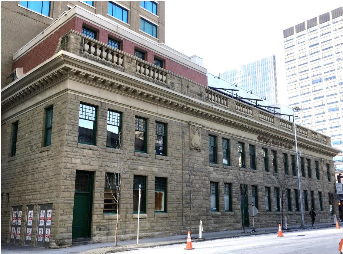
(Image 1.5: West façade, oblique from northwest)
