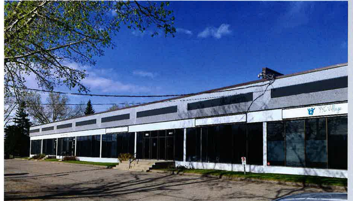
Looking North West
