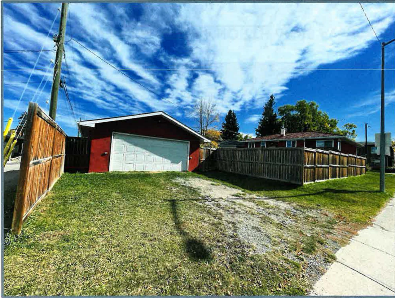
Detached garage accessed from 20 Street SW
