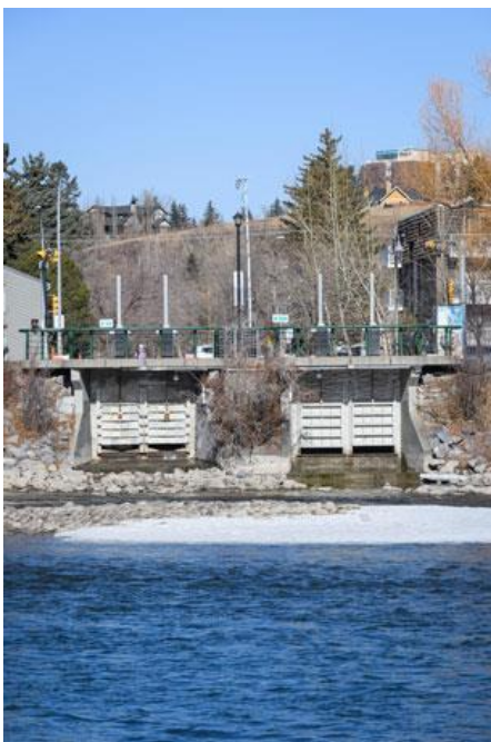
THE UPPER PLATEAU SEPARATION WILL PROVIDE AN EXPRESS ROUTE TO MOVE STORMWATER FROM THE COMMUNITIES ON TOP OF THE HILL DIRECTLY TO THE RIVER, BYPASSING SUNNYSIDE AND HELPING PREVENT FLOODING IN THE AREA.
