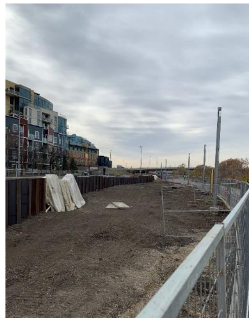
CONSTRUCTION ON THE DOWNTOWN FLOOD BARRIER BEGAN IN 2021
