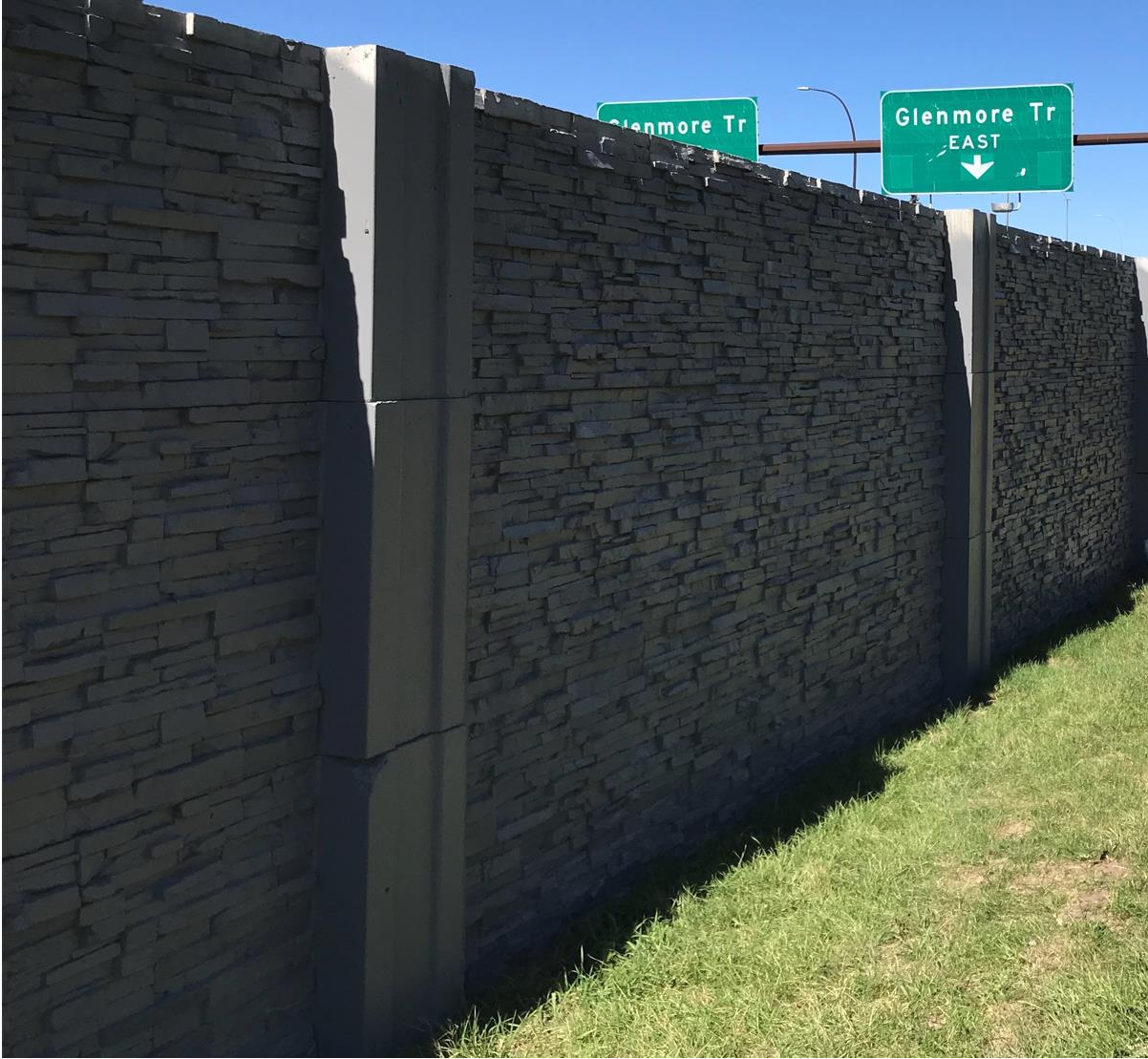
Example: 14 Street SW & Glenmore Trail SW. Pre-cast concrete w/ stack stone pattern
