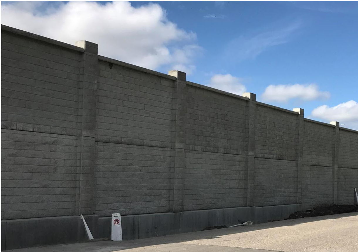
Example: Crowchild Trail SW & Glenmore Trail SW – precast concrete panel w/ brick lay patten
