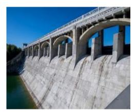
New higher gates at the Glenmore dam have doubled the reservoir's storage, providing valuable water supply and flood mitigation on the Elbow River.
