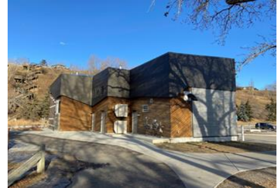
Community Drainage Improvements
