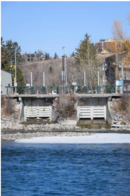
THE UPPER PLATEAU SEPARATION WILL PROVIDE AN EXPRESS ROUTE TO MOVE STORMWATER FROM THE COMMUNITIES ON TOP OF THE HILL DIRECTLY TO THE RIVER, BYPASSING SUNNYSIDE AND HELPING PREVENT FLOODING IN THE AREA.
