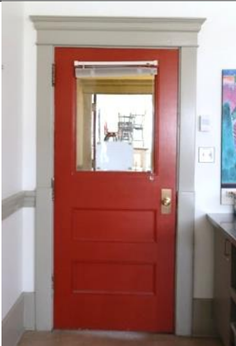
Image 3.4: Example of a paneled wooden door with single light
