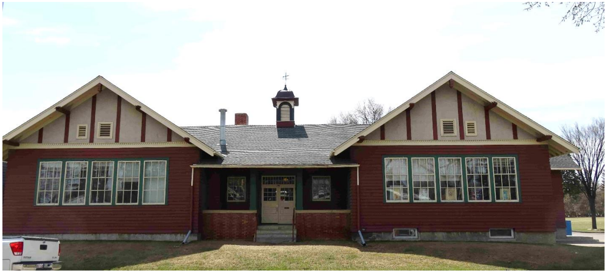
(Image 2.2: North façade)
