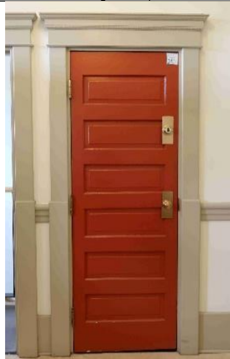
Image 3.5: Example of a paneled wooden door
