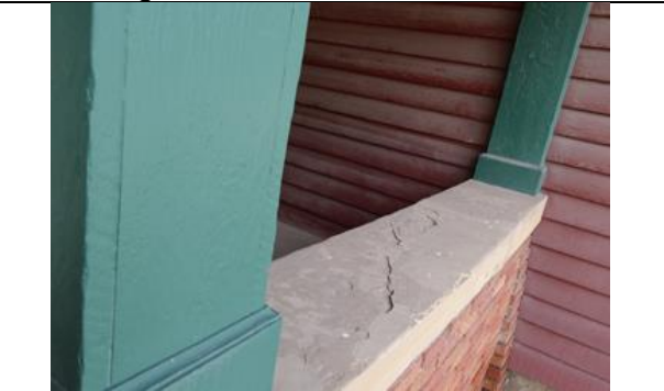
2.14: Example of sandstone capped balustrade
