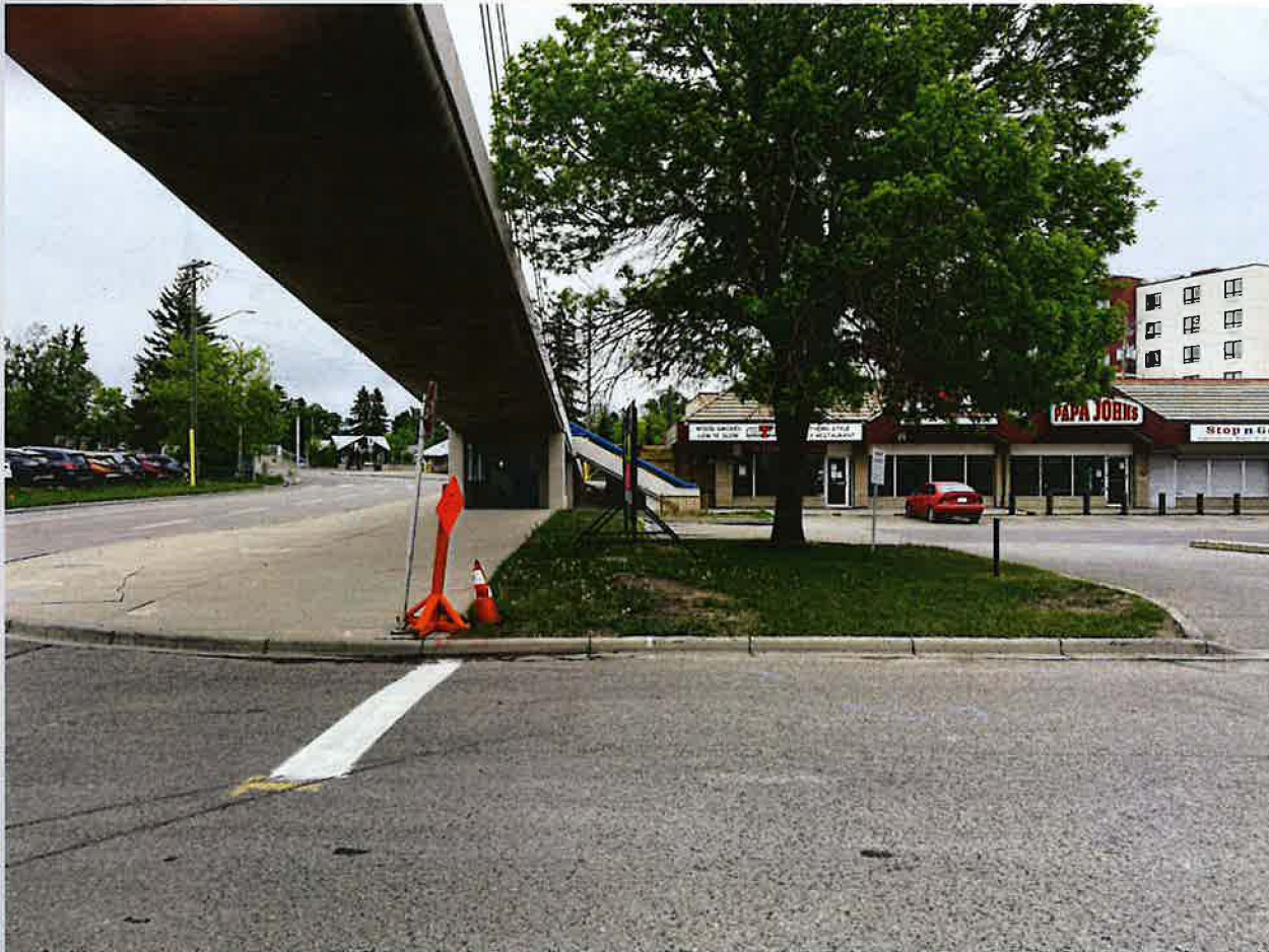
View of the site from 24 Street NW
