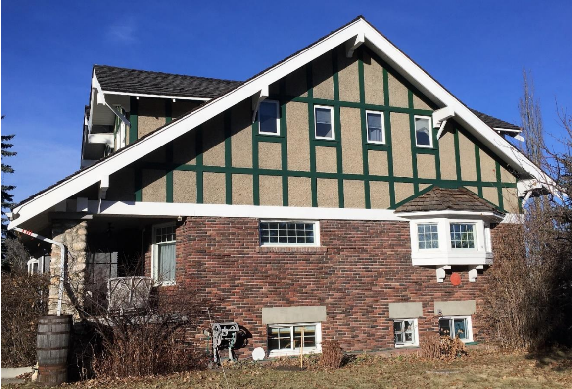
(Image 2.7: Southeast façade showing deeply pitched gable roof, front- and rear-facing cross-gables; heavy gable trim; deep eaves; exposed rafters; painted wood belt course, and fenestration)
