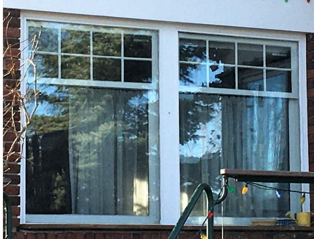
Image 2.13: Original double assembly of 8-over-one hung sash windows
