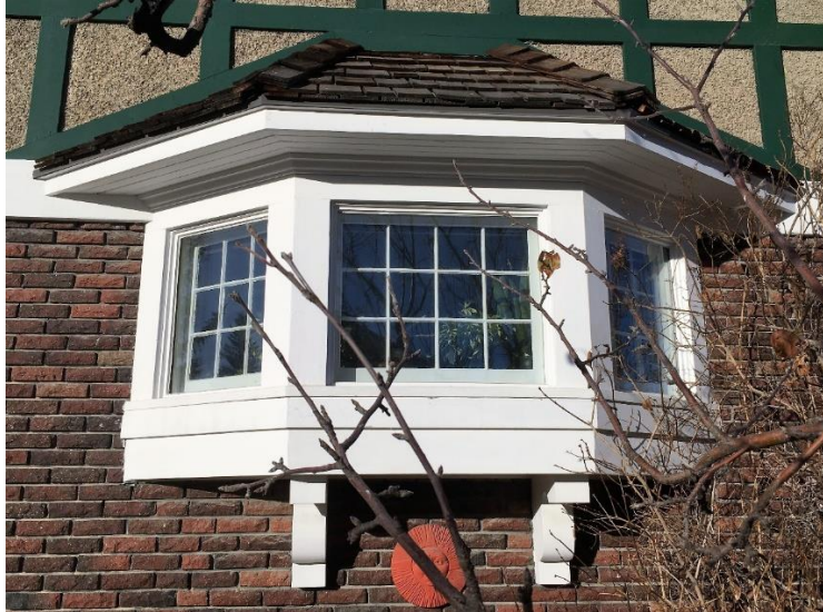
Image 2.12: Original canted bay window; hip roof, deep tongue-and-groove eaves; painted wood casings and moulded brackets
