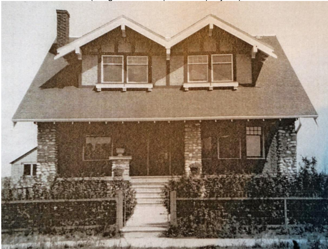
(Image 2.2: Historical image of Front (southwest) façade)
