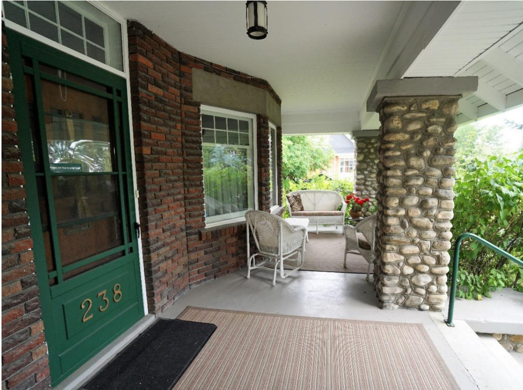
(Image 2.3: Veranda faced with clicker-brick facing in stretcher bond, pillars faced with fieldstone and mortar beading; tongue-and-groove eave; front entry with wood surrounds; 8-light transom and solid oak entrance door with 4 'gun-slit' windows with clear beveled glass)
