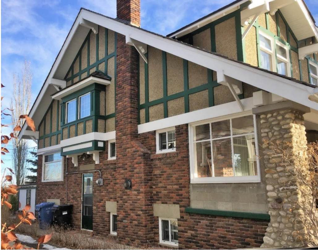
(Image 2.9: Northwest façade showing deep gable roof, front-facing cross-gable; heavy gable trim; deep eaves; exposed rafters; painted wood belt course and fenestration)
