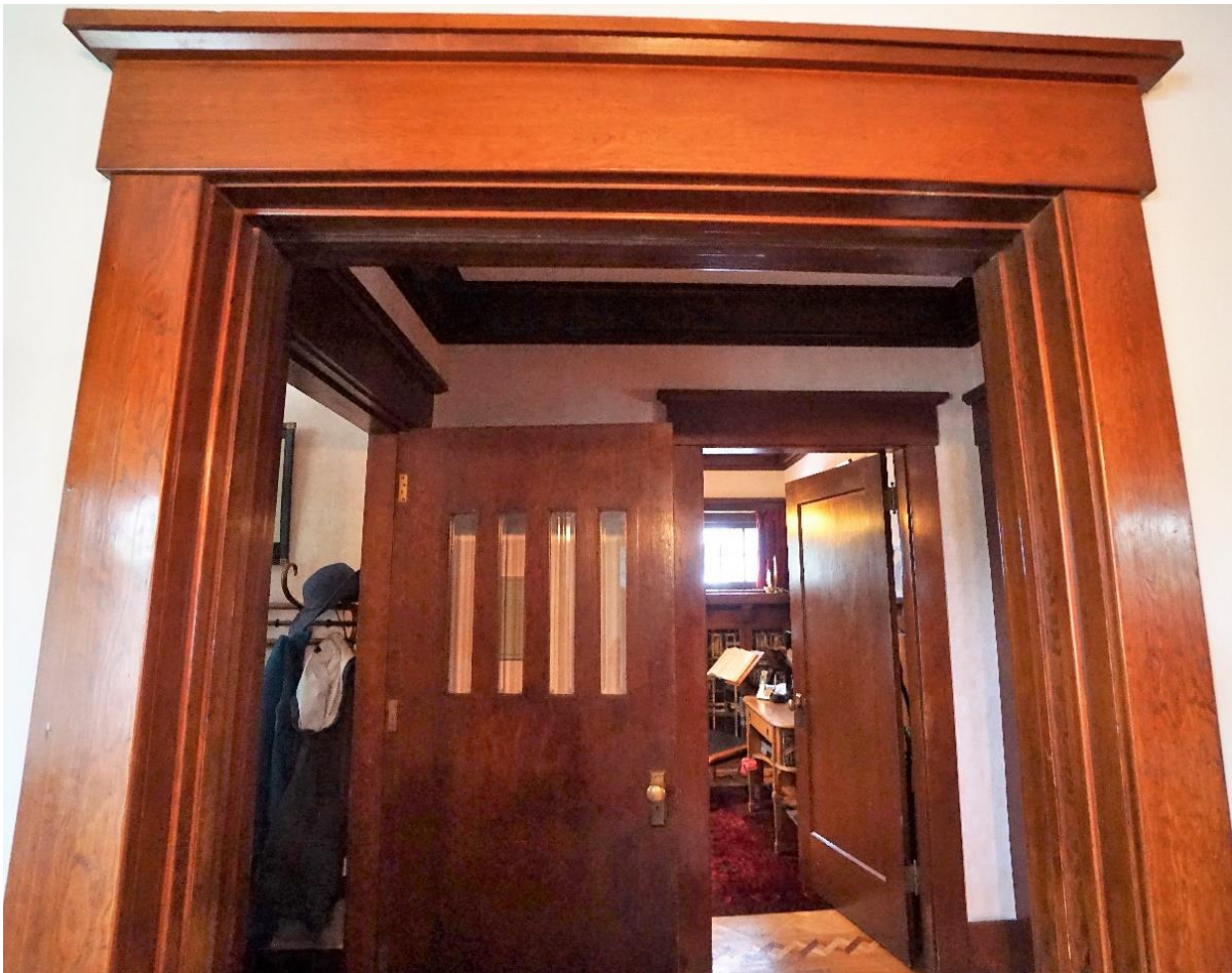
(Image 3.1: Wood door casings; crown moulding; extant oak parquet flooring)
