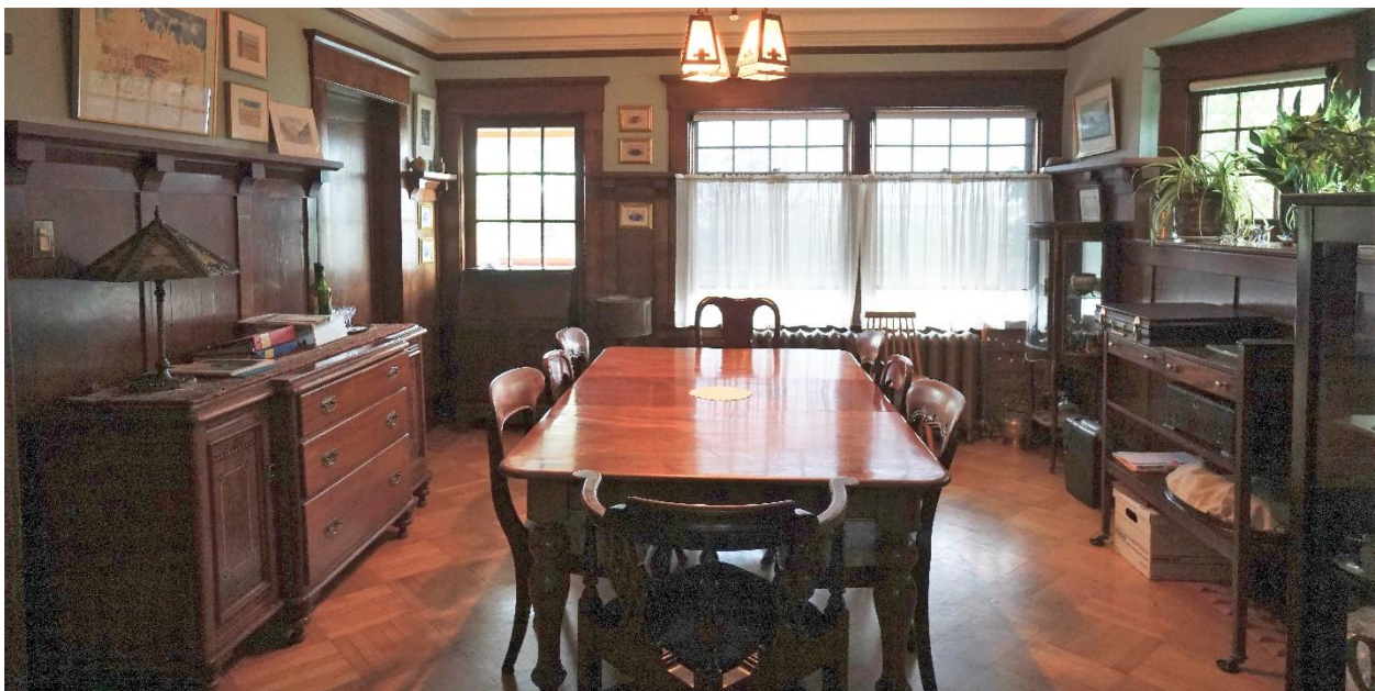
(Image 3.5: Door and window casings; panelled wainscoting topped by bracketed plate rails; oak parquet floor)
