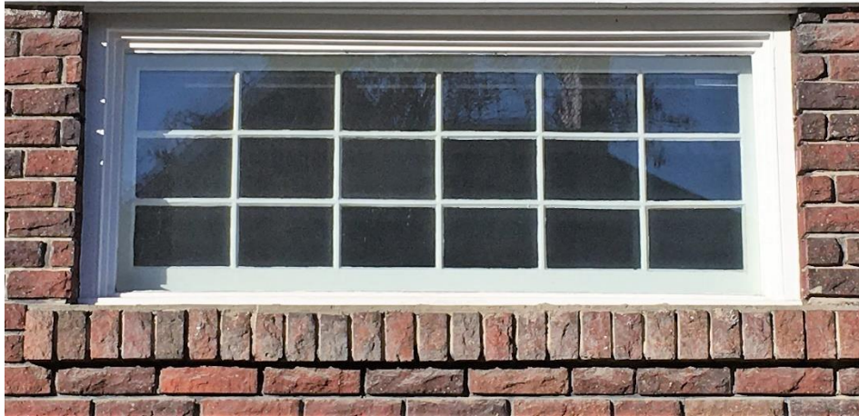
Image 2.11: Original fixed multi-light wood sash window
