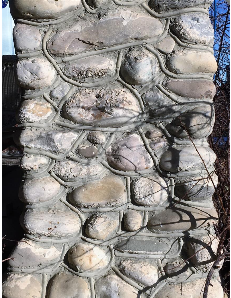
Image 2.6: Detail of fieldstone-clad pillar with mortar beading
