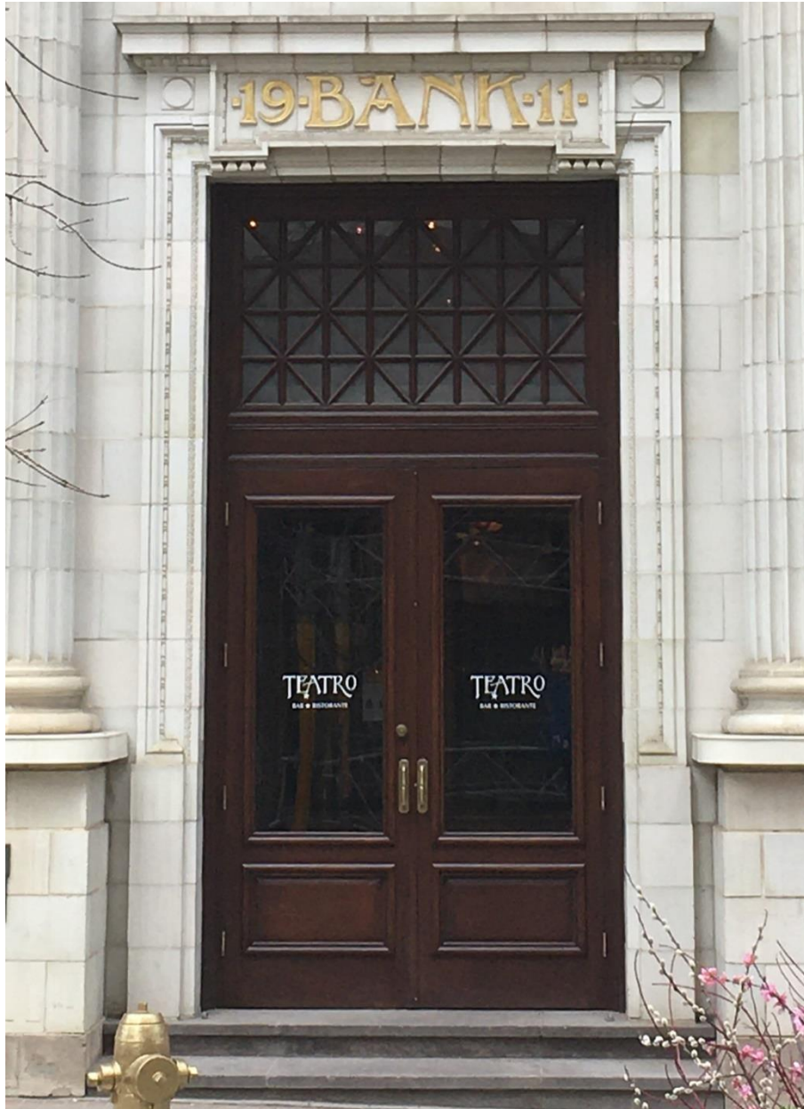
(Image 1.6: South entryway, decorative door surround '19 Bank 11' sign band, double oak doors with single lights with diamond wooden sash transom; granite door threshold)
