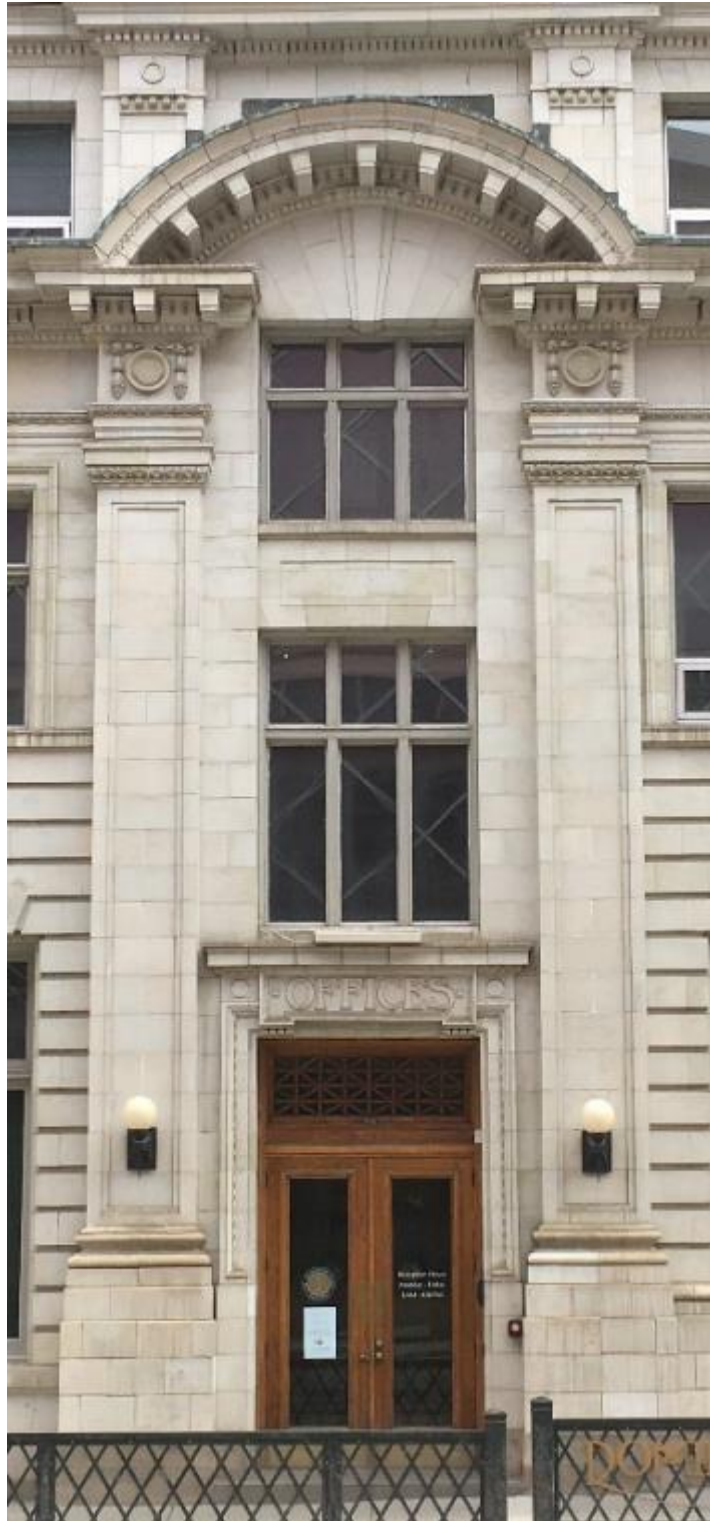
(Image 1.7: West façade, main entryway with two storey surround with pilasters; arched hood at cornice)
