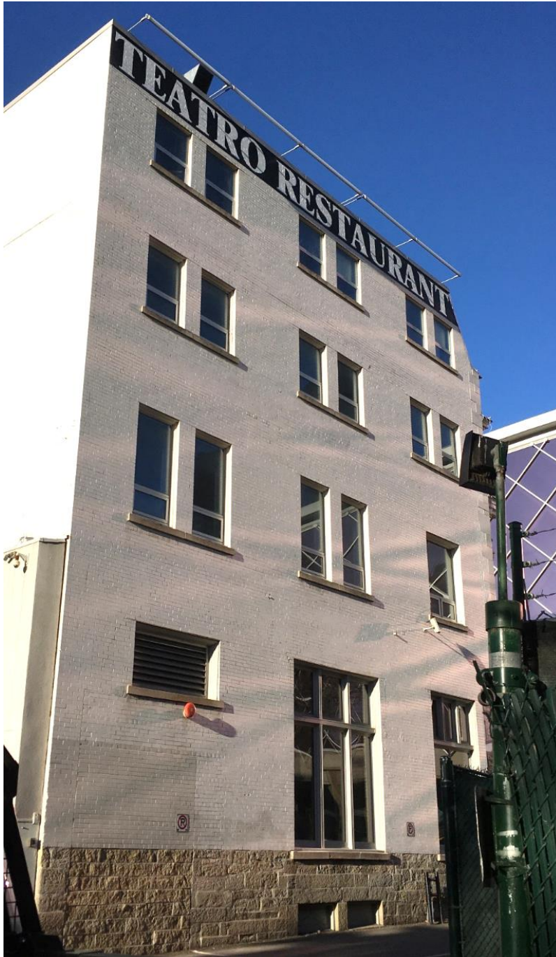
(Image 2.1: North façade with square cut ashlar sandstone and brick wall in common bond)
