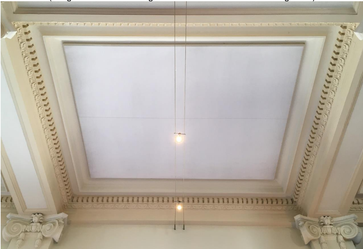
(Image 2.6: Detail of coffered insets with dentil and leaf detailing)
