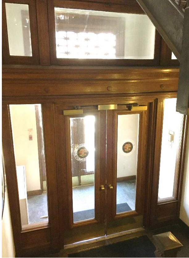
(Image 2.4: Double oak doors with transom and side lights at west entryway, terrazzo floor in outer vestibule)
