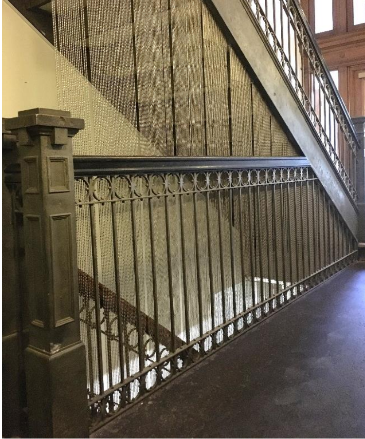
(Image 2.2: Original steel staircase, balustrade and newel post in west inner vestibule)
