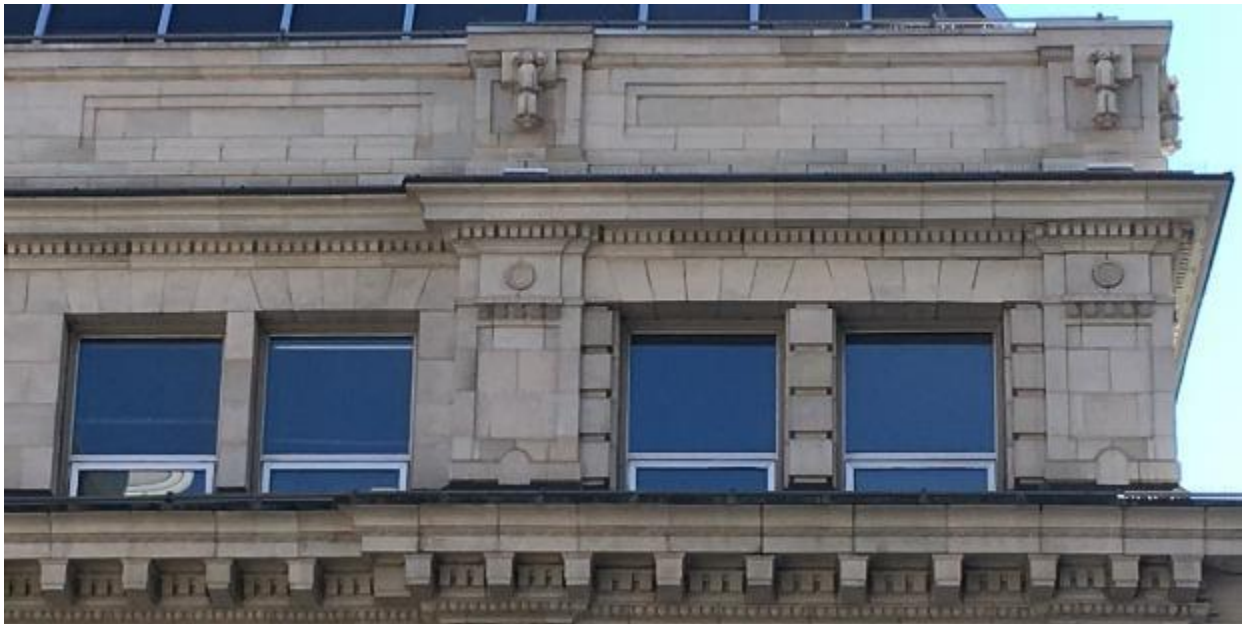
(Image 1.5: Detail of large and small cornices, pilasters in terracotta units decreasing in scale towards roofline, and floral and shield detailing)
