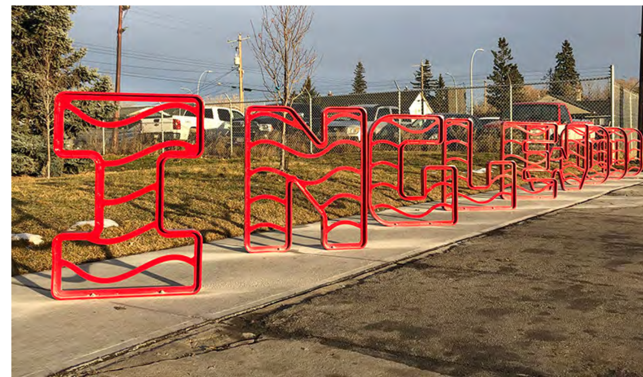
Custom 'Inglewood' bicycle rack installed along the project site's south edge
