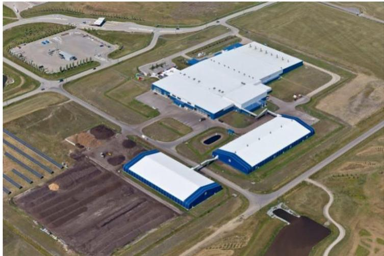
operation of composting facilities. The open procurement resulted in a facility capable of processing 100,000 tonnes per year of food and yard waste and 45,500 tonnes per year of biosolids.
