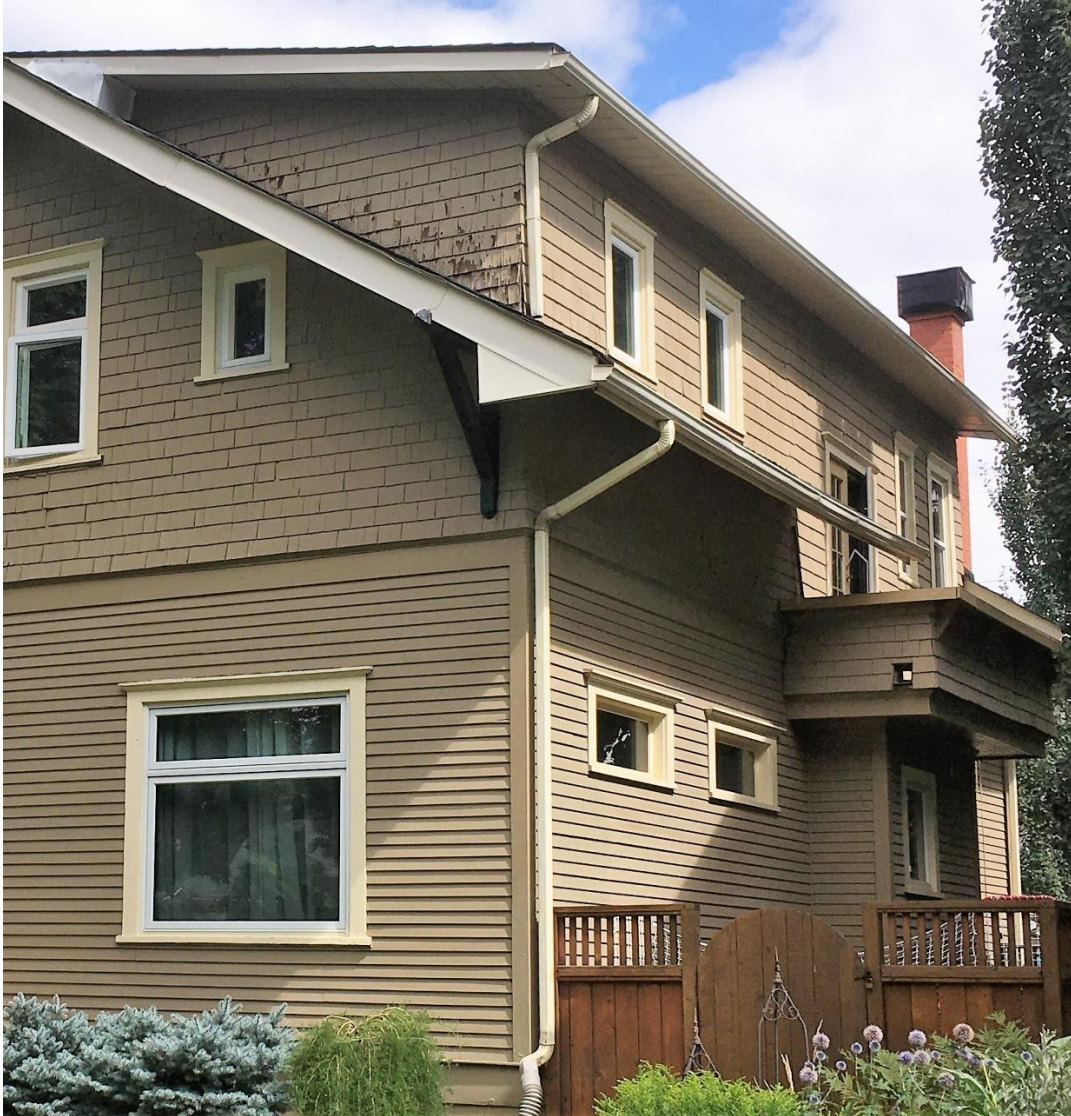
(Image 2.5: South façade with shed roof over dormer; upper level balcony, three-sided bay)
