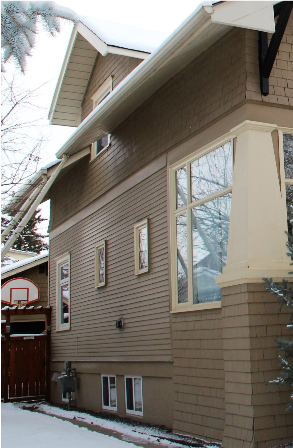
(Image 2.4: North façade with gable over north facing dormer; water table with drip mould and examples of flared, wood shingle corners)
