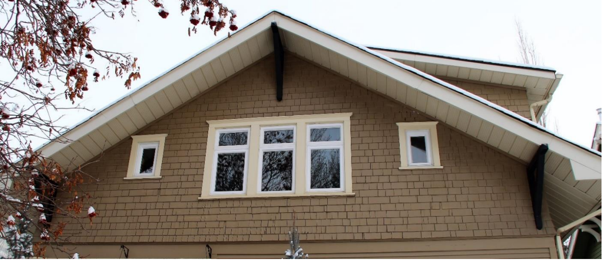
(Image 2.2: Front gable with deep eaves; triangular brackets; shed roof over south facing dormer)
