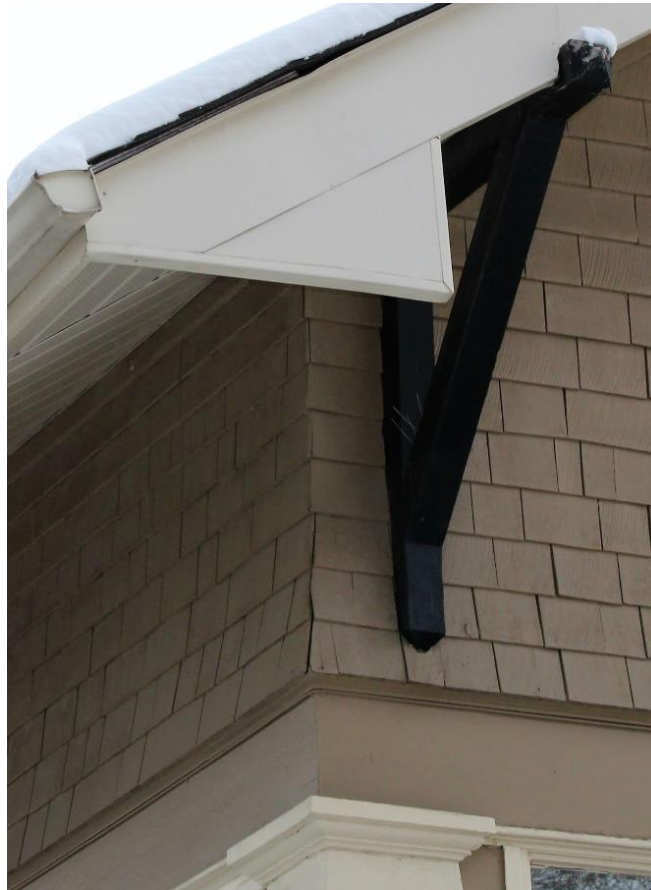
(Image 2.3: Example of wood shingles with flared corners on the upper storey and triangular brackets)
