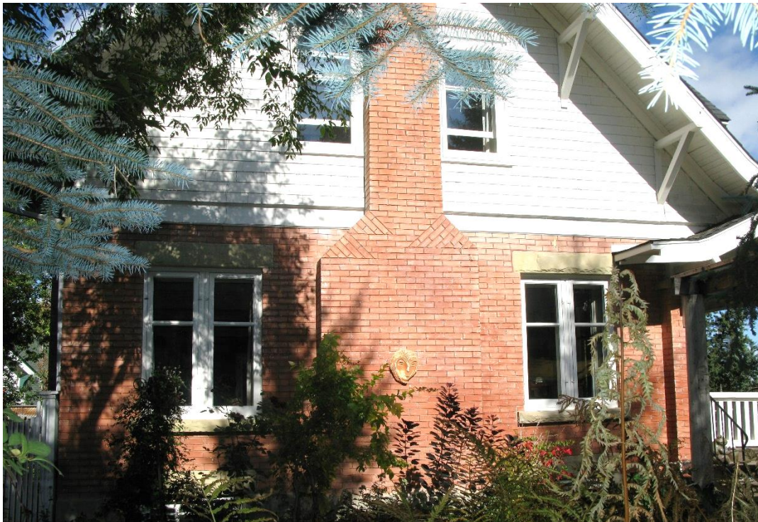
(Image 2.3: Southeast façade)
