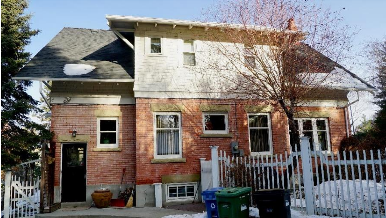
(Image 2.4: Southwest façade)
