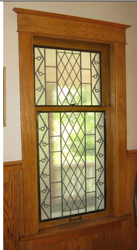
Image 3.2: Example of 1st storey original moulded oak window casing
