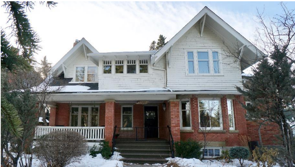
(Image 2.1: Northeast façade)
