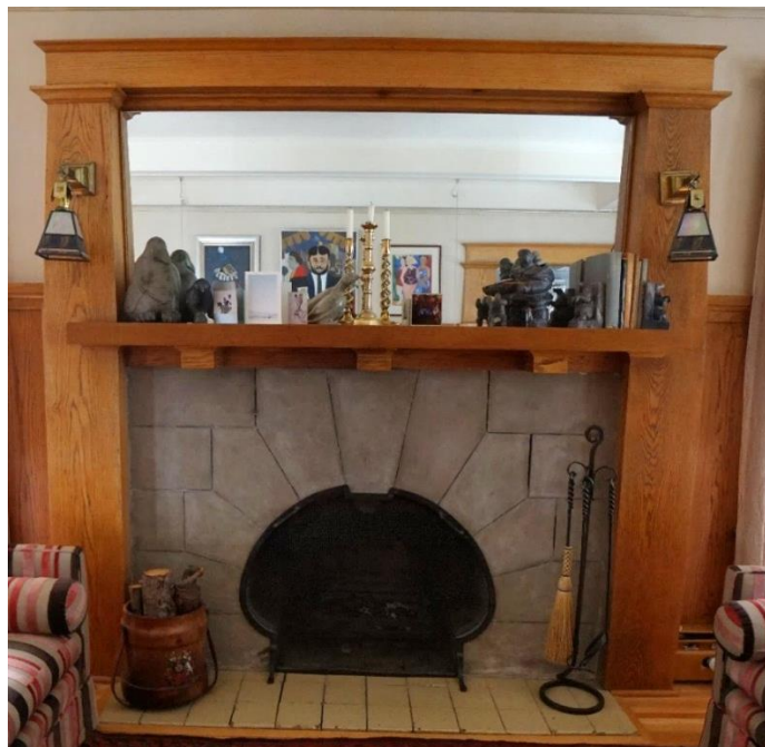
(Image 3.8: Round-arch stone fireplace with keystone; molded oak mantelpiece, bracketed oak mantelshelf; square glazed hearth tiles)
