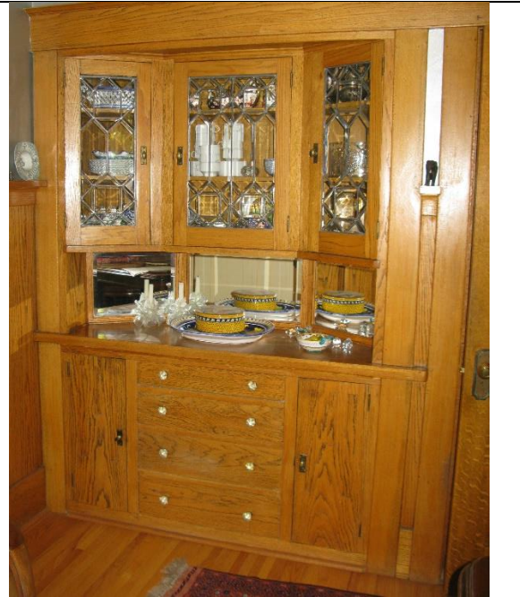
Image 3.7: Dining room built-in oak cabinet with leaded glass fronts in geometric patterns
