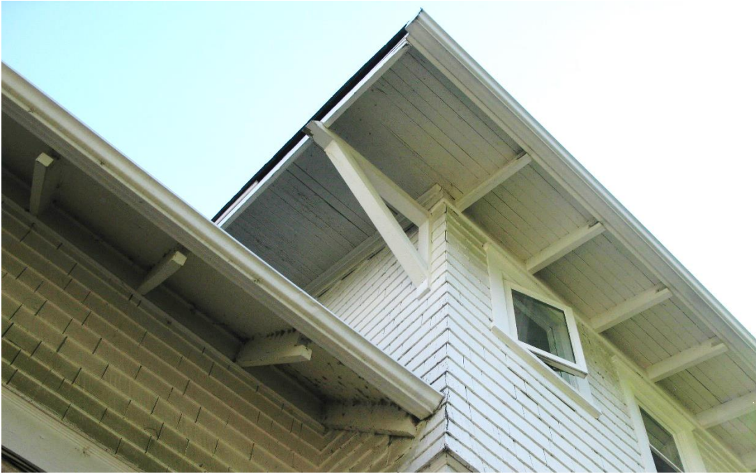
(Image 2.6: Examples of deep eaves with tongue-and-groove soffits; painted-wood triangular roof brackets; exposed rafters with notched ends)
