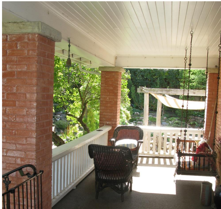
(Image 2.7: Detail of verandah with plain porch balustrade and red brick porch posts with plain sandstone caps)
