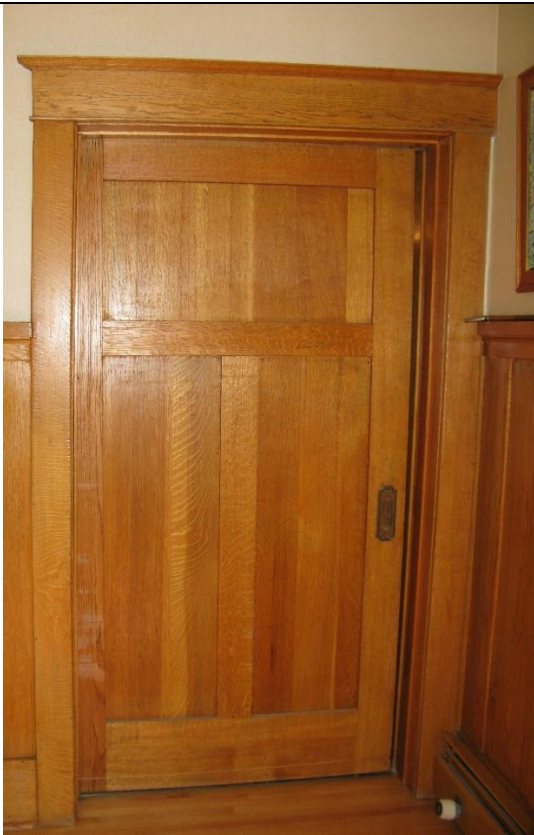
Image 3.1: Example of 1st storey original moulded oak doorway casing, baseboards, and panelled oak door
