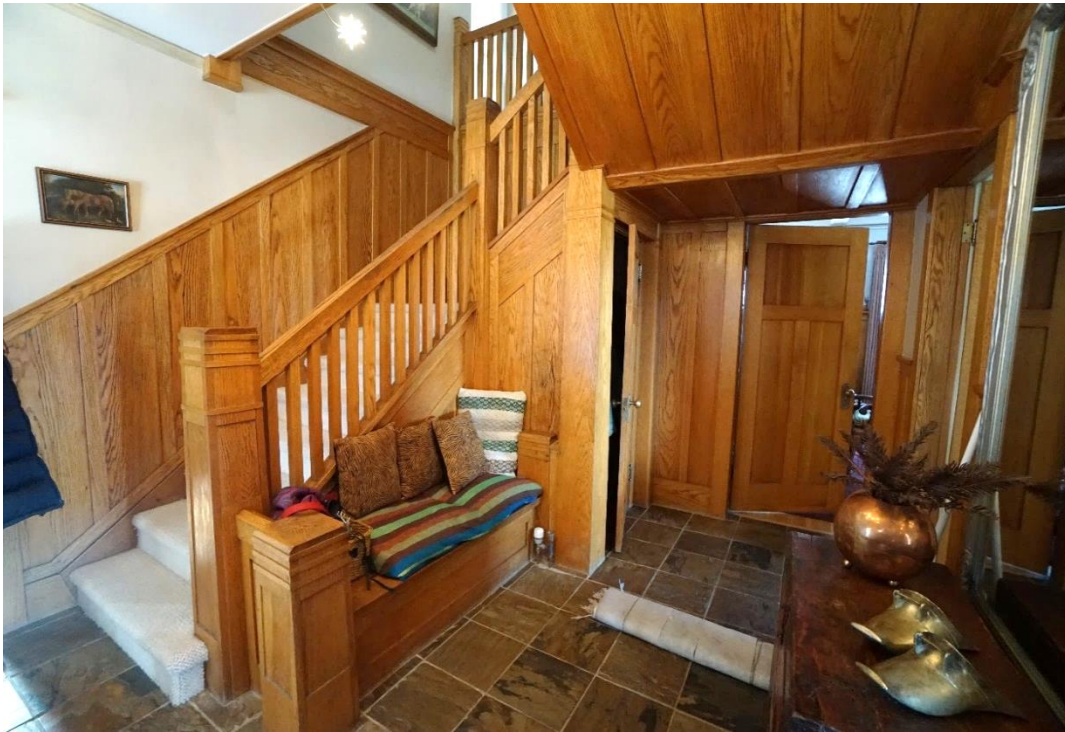
(Image 3.3: Oak closed-string, open-well staircase with oak plain railing, square panelled newel posts with horizontal banding, flat caps; foyer oak wall and ceiling paneling; oak storage bench)
