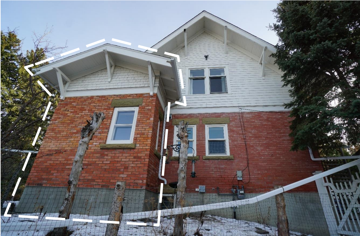
(Image 2.2: Northwest façade. Dashed outline indicates the corner single storey extension built ca. 2013 that, while sympathetically designed, is not regulated)
