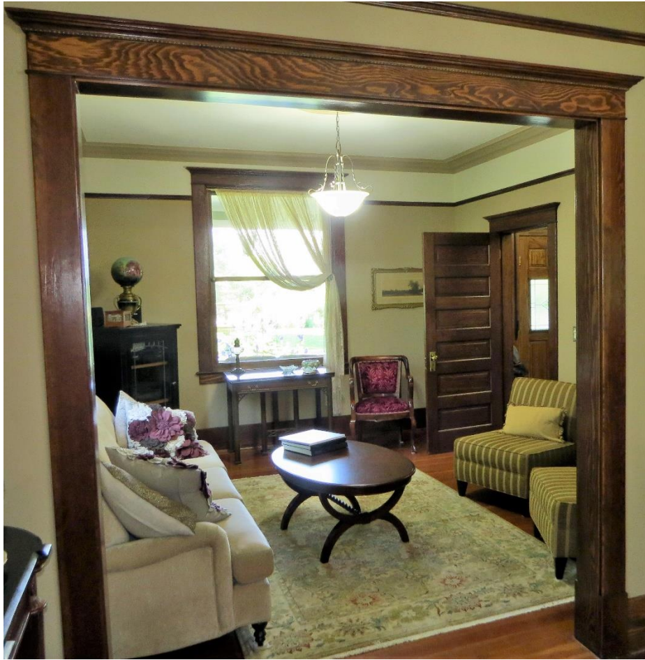
(Image 4.3: Example of wood trim including door and window casings, living room arch, typical six panel door plaster moulding around edge of living room ceiling)
