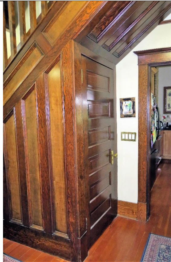
Image 4.2: Main floor staircase wood panelling; typical six panel door.
