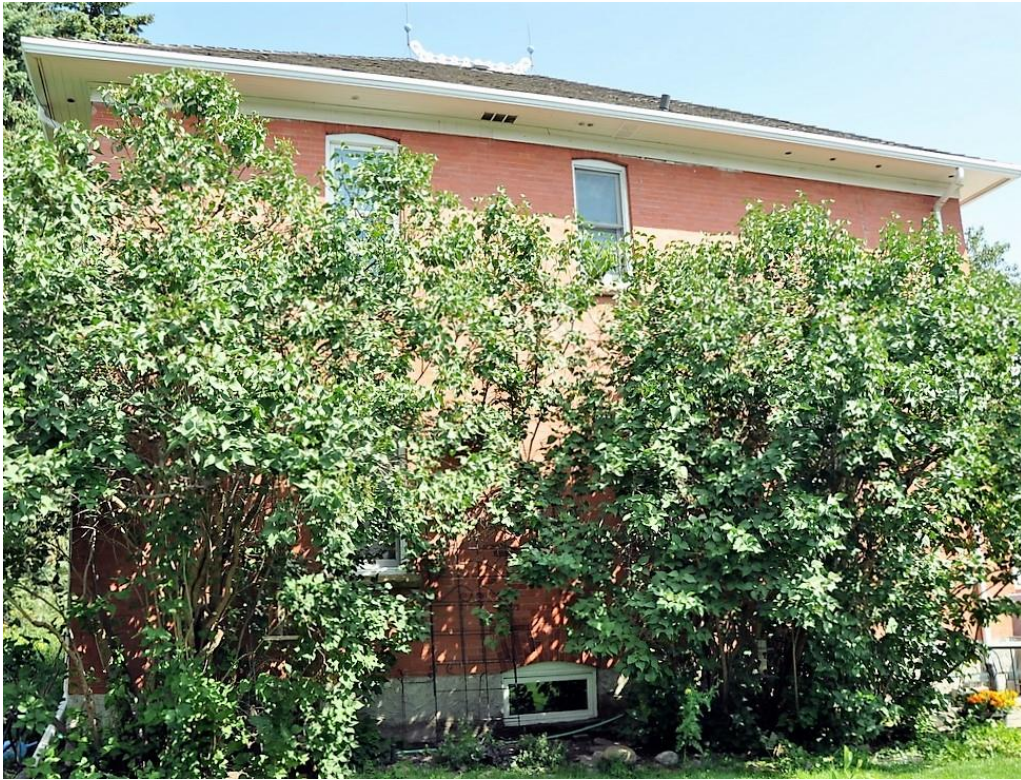
(Image 2.6: West façade.)
