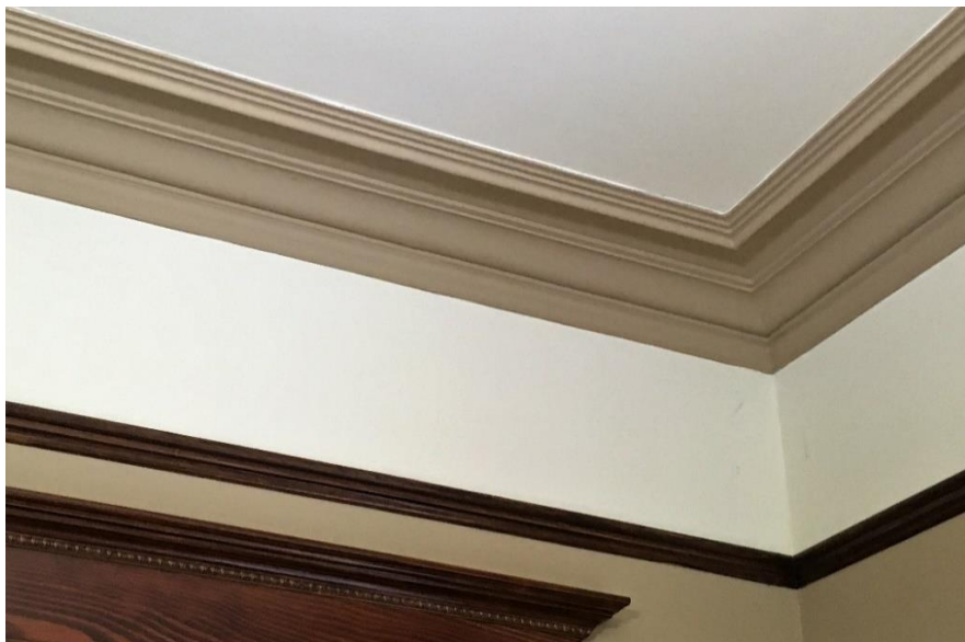
(Image 4.4: Detail of plaster moulding around edge of living room ceiling)
