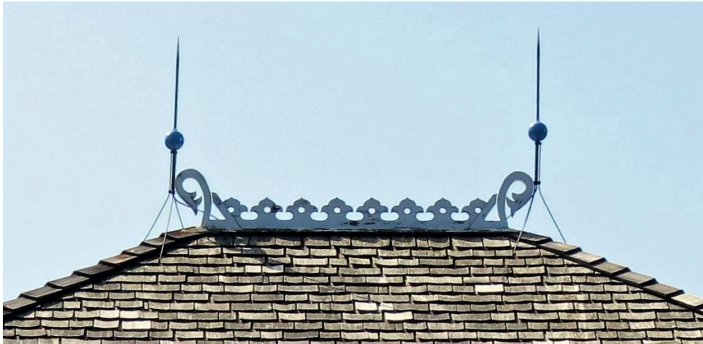
(Image 3.1: Detail of roof cresting and lightning rods)
