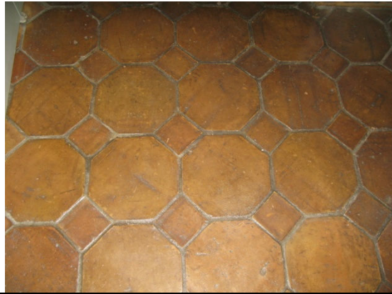
(Photo 6.18: an example of the Mexican clay-tile flooring)
