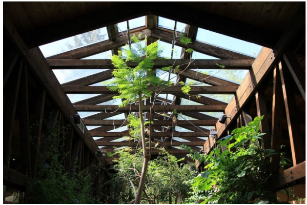
(Photo 5.2: the glass skylight /greenhouse roof spanning the central courtyard –view from interior)
