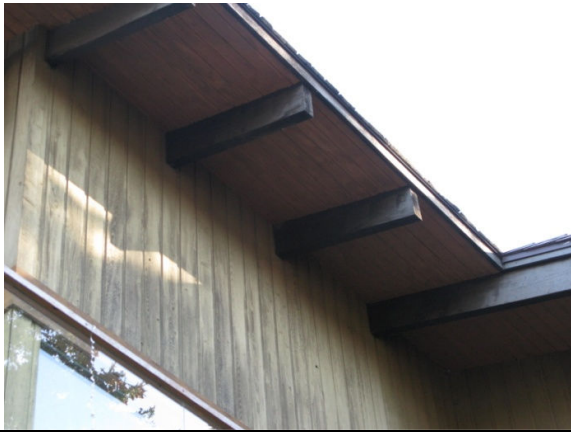
(Photo 5.1: an example of the wooden soffits and exposed rafters)
