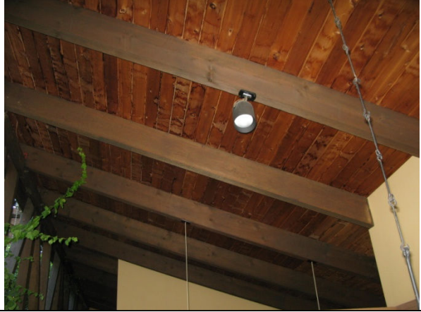
(Photo 6.14: detail view of the wooden tongue-and-groove ceiling and exposed rafters)
