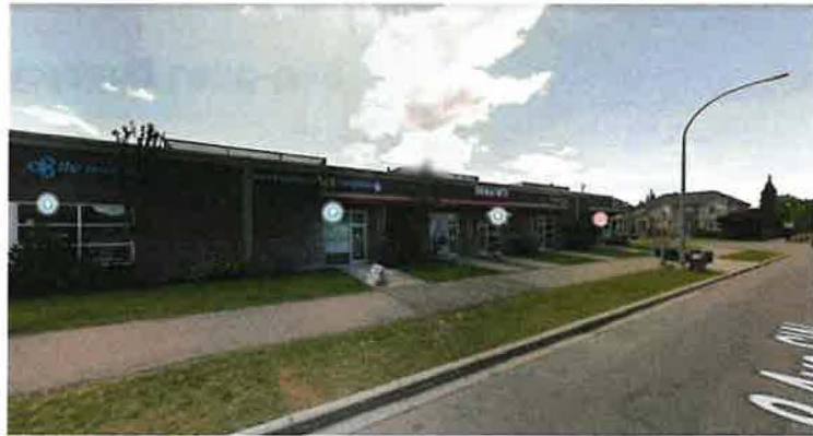
6 View of 9 Ave SW looking West
