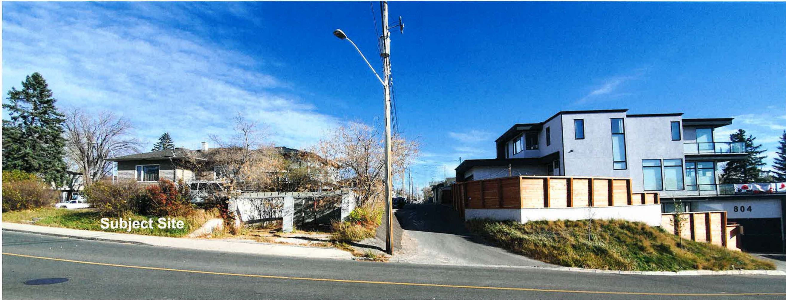
View of the subject site, looking east
