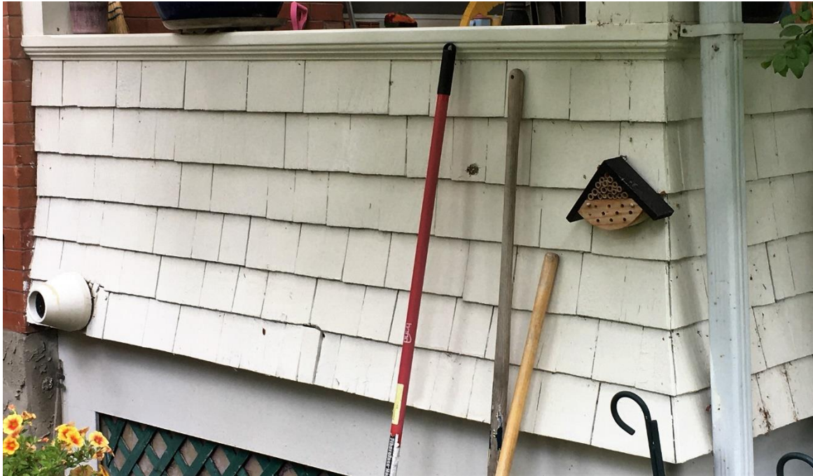
(Image 2.4: Detail of wood shingle clad verandah with flared, wood shingle corners)
