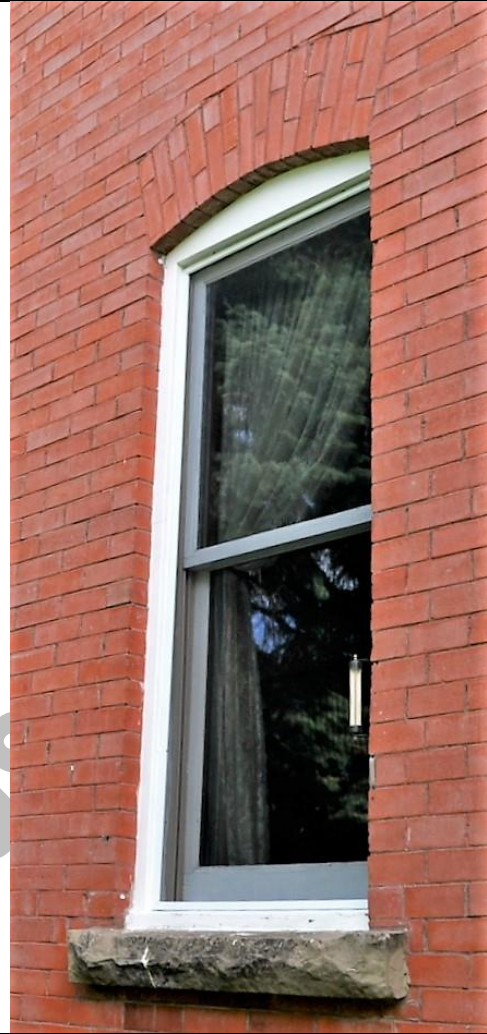
Image 2.3: Detail of typical fenestration and hung profile
