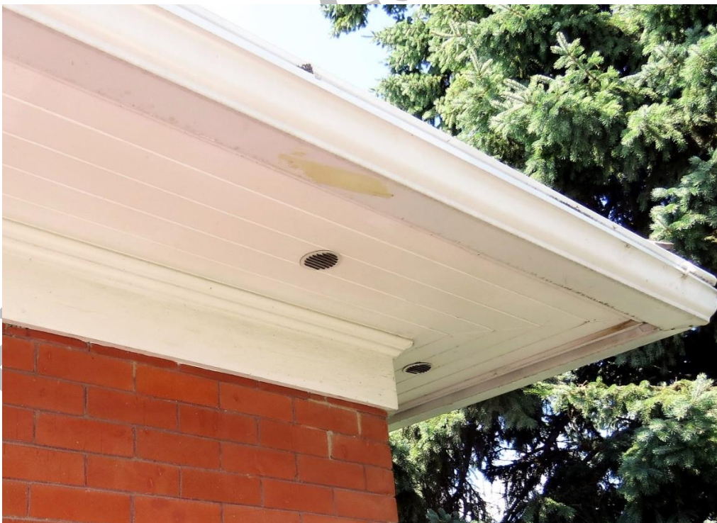
(Image 3.2: Detail of eave; wooden tongue-and-groove soffits, wooden fascia and moulded frieze)
