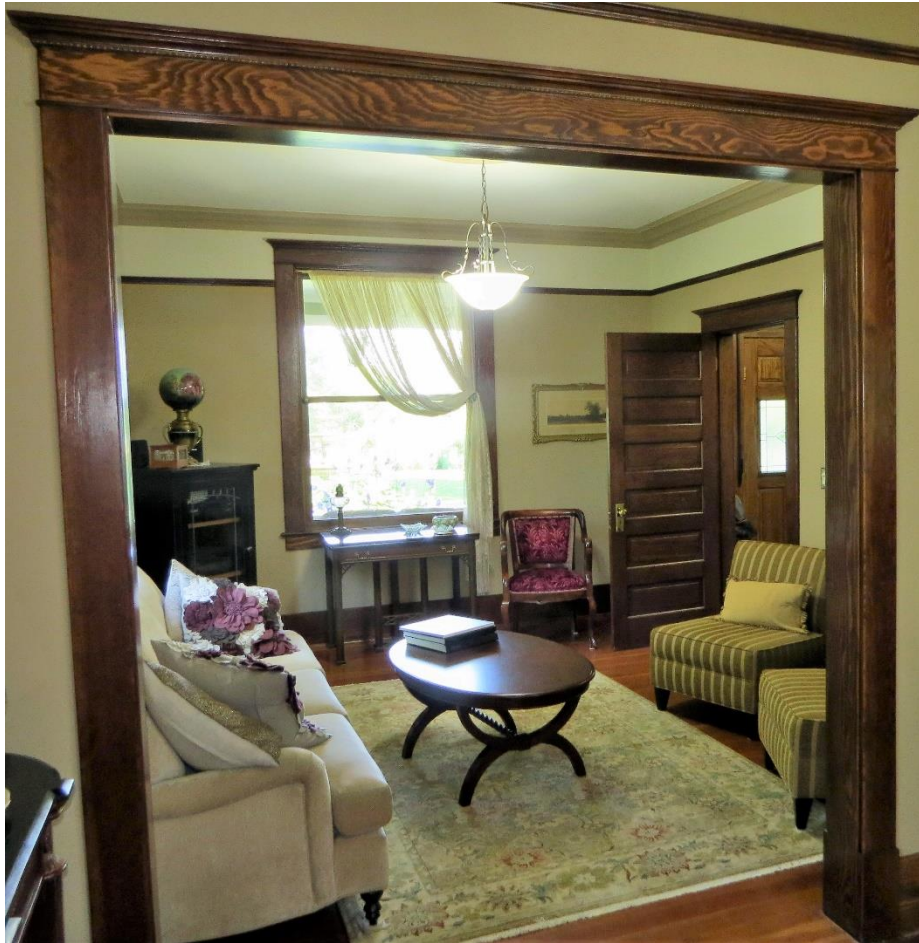
(Image 4.3: Example of wood trim including door and window casings, living room arch, typical six panel door plaster moulding around edge of living room ceiling)
