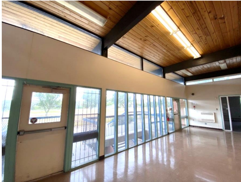
(Image 3.1: Open foyer at upper storey with clerestory windows, glulam beams and wood-paneled ceiling)
