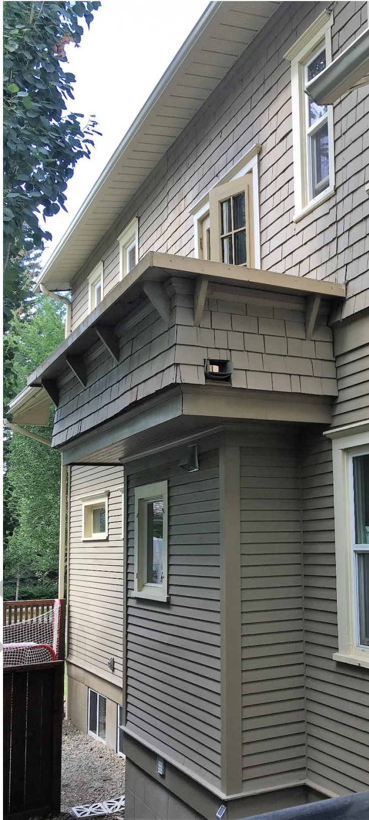
(Image 2.6: Detail of three-sided bay, upper level balcony with wood shingle cladding, closed balustrade; wood moulding and fascia; tongue-and-groove soffit)
