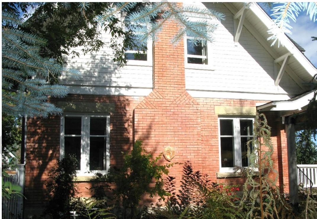
(Image 2.3: Southeast façade)
