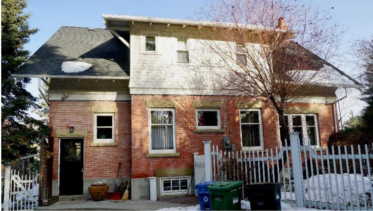
(Image 2.4: Southwest façade)
