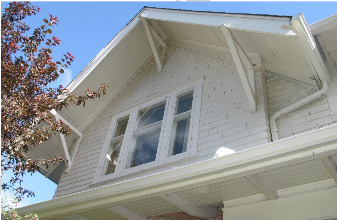
(Image 2.5: Examples of deep eaves with tongue-and-groove soffits; painted-wood triangular roof brackets; fascia with notched ends)
