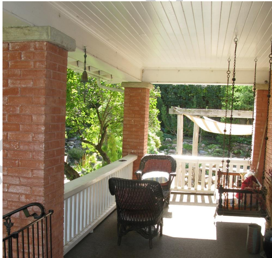
(Image 2.7: Detail of verandah with plain porch balustrade and red brick porch posts with plain sandstone caps)
