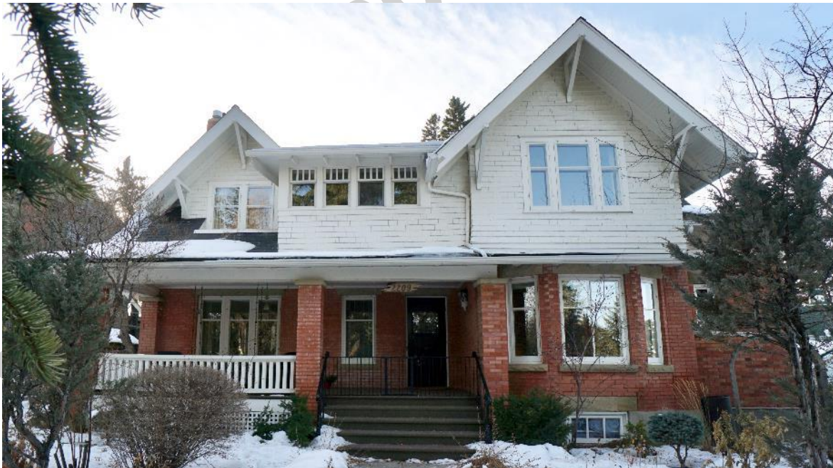
(Image 2.1: Northeast façade)
