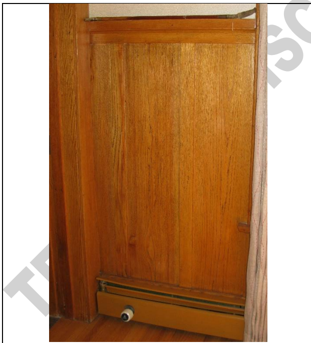
Image 3.4: Example of living room oak wall panelling
