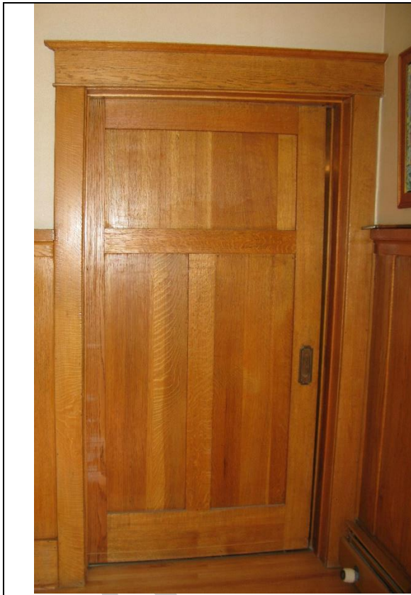
Image 3.1: Example of 1st storey original moulded oak doorway casing, baseboards, and panelled oak door
