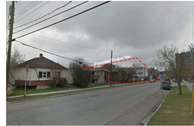
STREET VIEW LOOKING EAST (FRONT)
