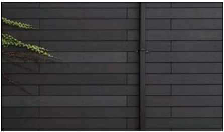
09 GFRG SLATS (CURVED WALL & L- FRAME) GREY TONES
