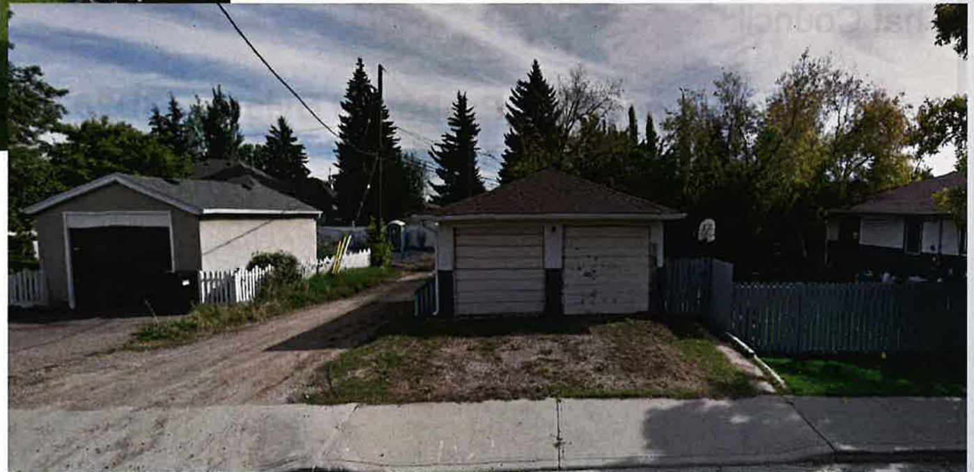
East side showing existing driveway
