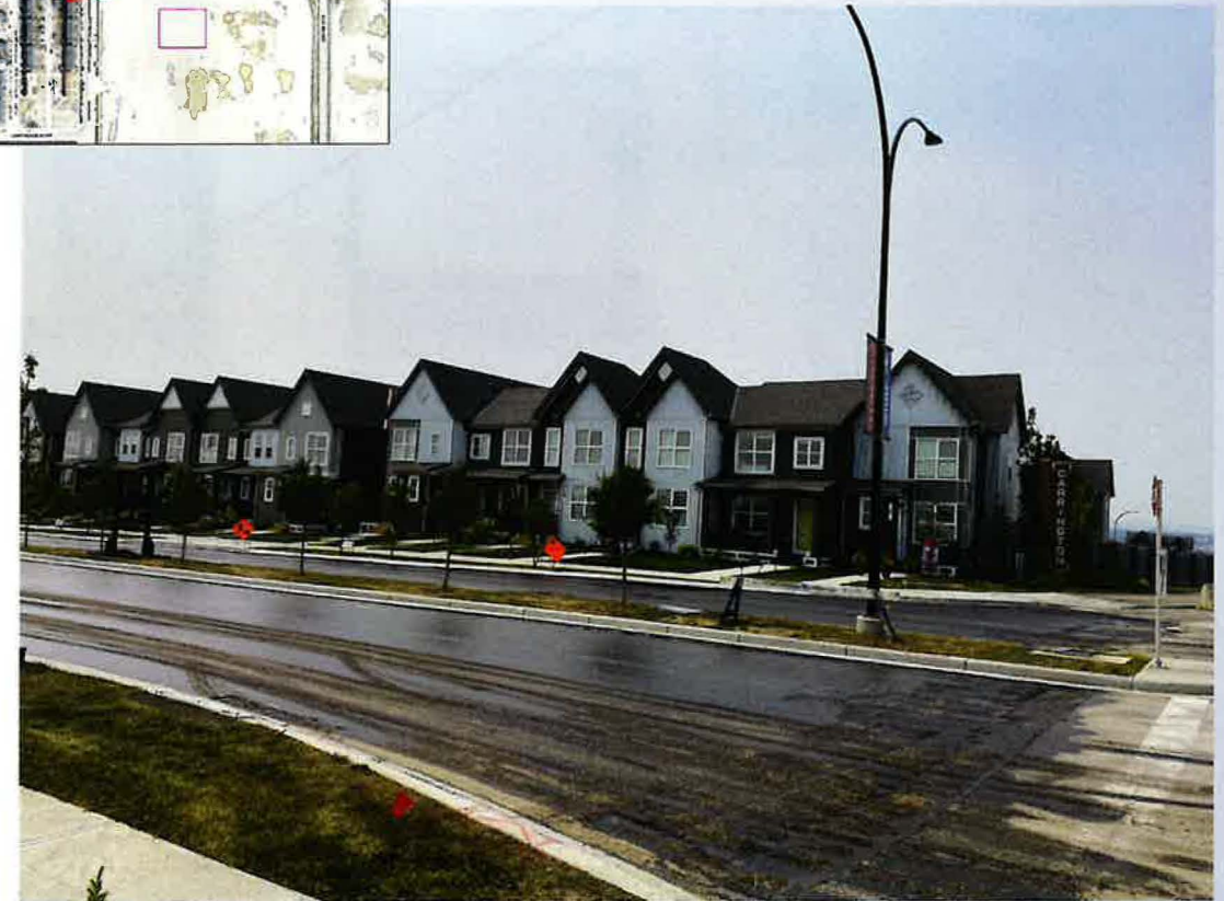
Existing residential development, west of Carrington Boulevard NW
