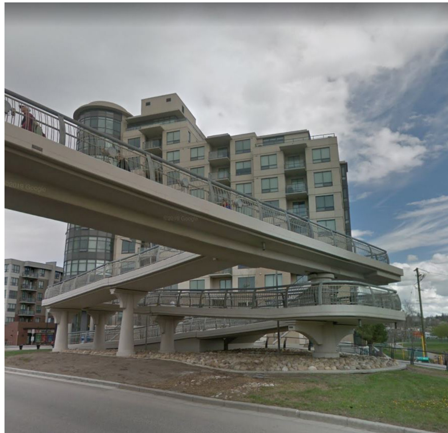
Existing 2005 north LRT pedestrian bridge and ramp
