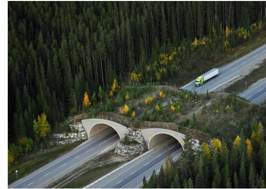
Banff Animal Crossing Year: 2006 Span: 80m Width: ~50m Total Project Cost: $4,000,000 Linear Cost: $50,000/m * Animal crossing bridge, landscape bermed up to structure
