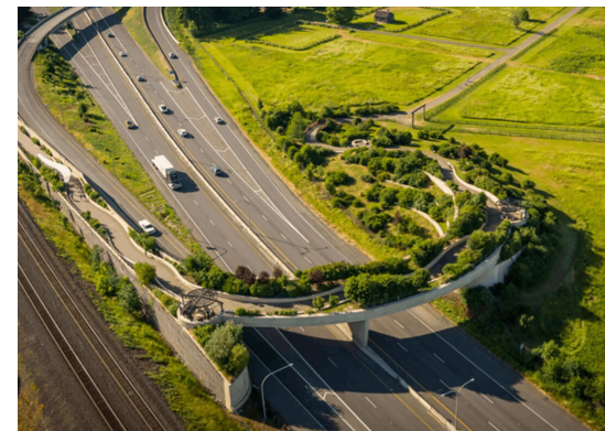
Vancouver, WA Land Bridge Year: 2006 Span: 60m Width: 12m Total Project Cost: $12,000,000 USD Linear Cost: $200,000 USD/m * Pedestrian footbridge, includes ramping to bridge
