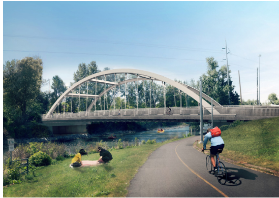
9 Ave S.E. Bridge Year: Under Construction Span: 65m Width: ~24m Total Project Cost: $23,000,000 Linear Cost: $353,847/m * Vehicular bridge, no additional ramping to bridge
