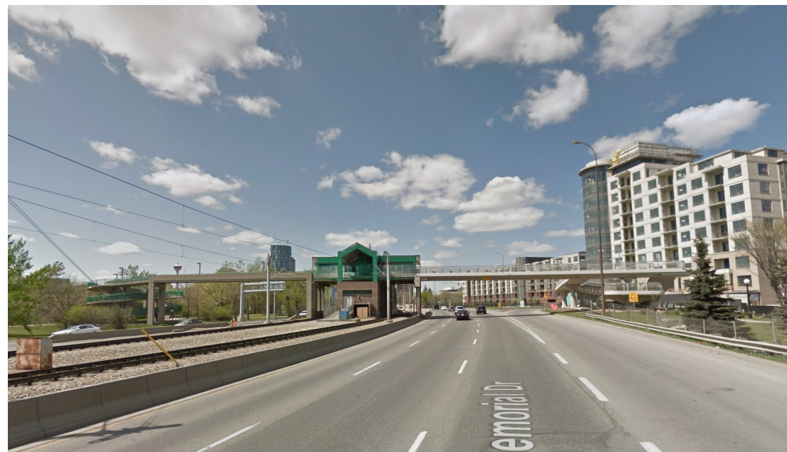
View along Memorial Dr N looking west
