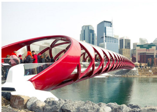
Peace Bridge Year: 2010 - 2012 Span: 130m Width: 6.2m Total Project Cost: $25,000,000 Linear Cost: $192,308/m * Pedestrian footbridge, no additional ramping to bridge
