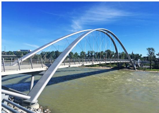
George C. King Bridge Year: 2012-2014 Span: 190m Width: Varies ~7.5m - 10.5m Total Project Cost: $25,000,000 Linear Cost: $131,579/m * Pedestrian footbridge, no additional ramping to bridge
