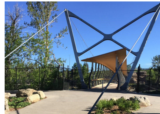
Calgary Zoo Bridge Year: 2018 Span: 60m Width: ~3m Total Project Cost: $3,000,000 Linear Cost: $50,000/m * Pedestrian footbridge, no additional ramping to bridge
