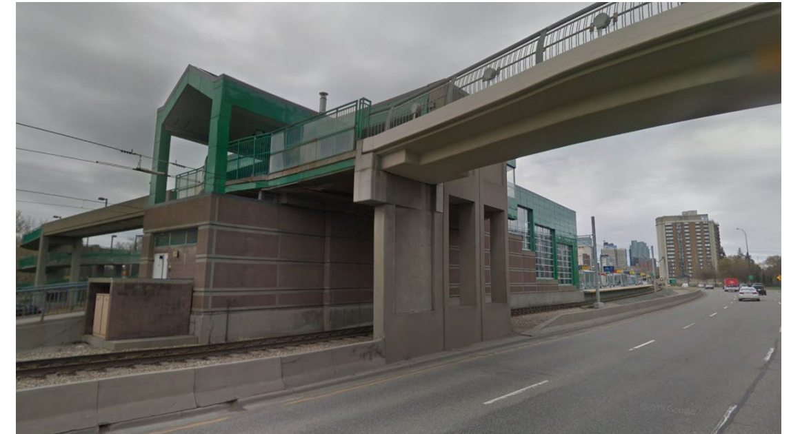
North side of station from Memorial Drive NE- existing structure infilled to meet current code requirements as part of station upgrade
