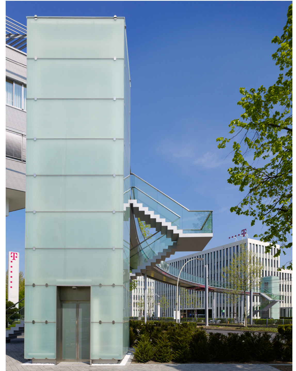
Exterior elevators can be designed to withstand extreme weather but are costly from an installation and operation and maintenance perspective.
