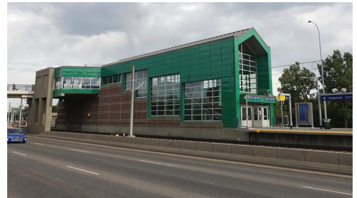
Station entrance and platform
