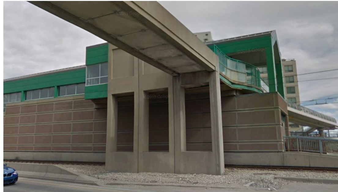
South side of station from Memorial Drive NE
