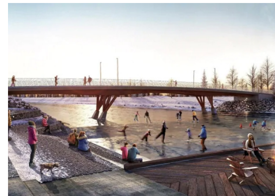
Jaipur Bridge Year: N/A Span: 60m Width: 6m Total Project Cost: $9,600,000 Linear Cost: $160,000/m * Pedestrian footbridge
