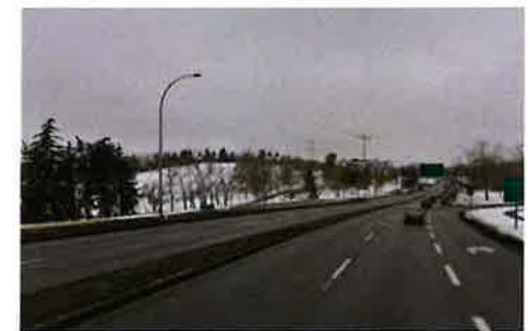
16 Avenue NW (TransCanada Highway) looking east.
