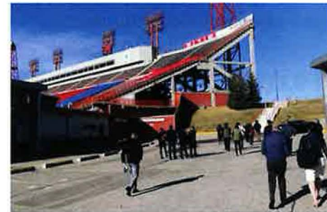
Site Walk Photo • South end of stadium moving east
