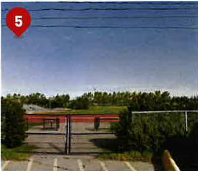
Central portion of the site, looking north towards the existing outdoor track.
