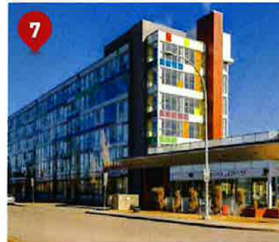
2520 Capitol Hill Crescent NW | Mid-rise
