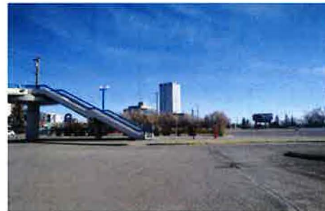
Site Walk Photo • East side of site pedestrian bridge
