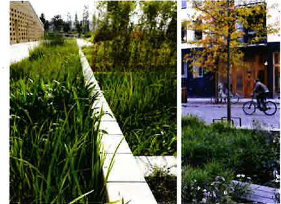
1. Engineered rain garden median
