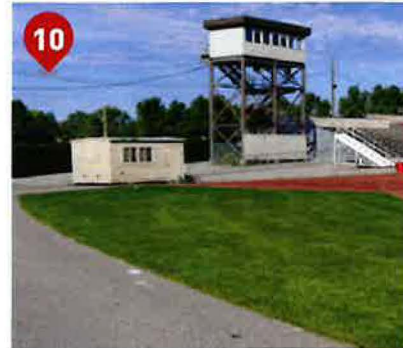
Central portion of the site looking east from the existing outdoor track
