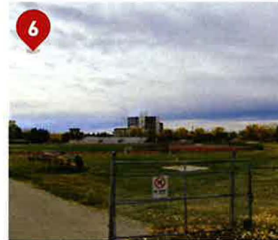
North side of the outdoor track, looking southwest
