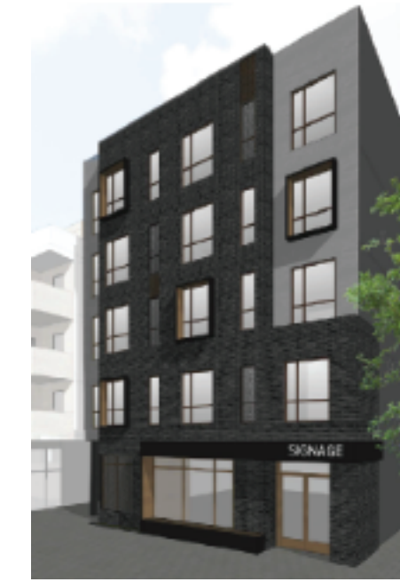
218 19 St NW M-U1f3.3h19 (24 Units, residential) In DP stage
