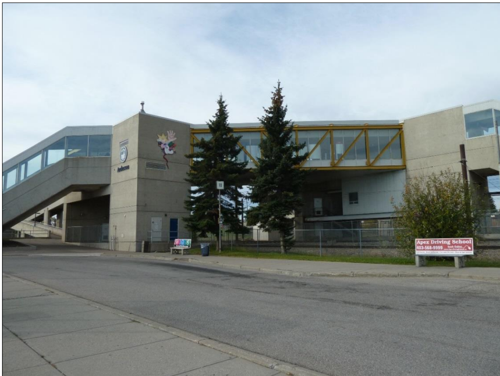
Figure 2: Anderson Station LRT Pedestrian Bridge -North Side View
