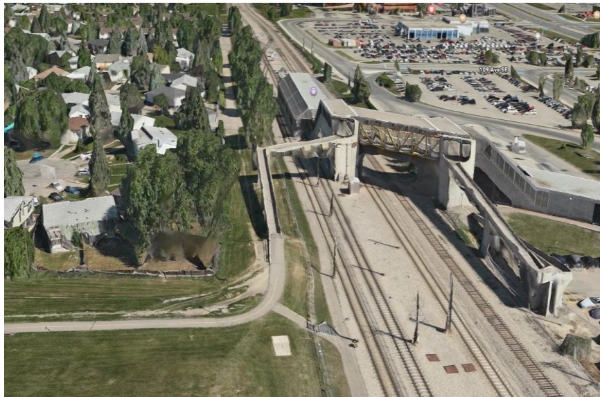
Figure 1: IMAGE OF EXISTING BRIDGE
