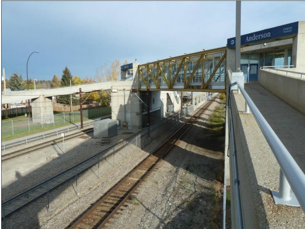
Figure 1: Anderson LRT Station Pedestrian Bridge – South Side View
