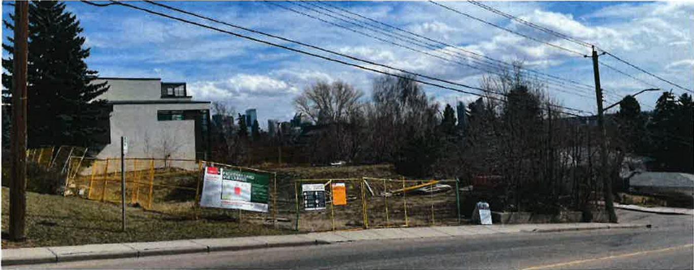
LOOKING SOUTHEAST FROM 19 STREET NW
