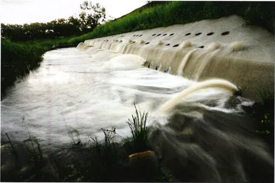
Photo source: https://www.csla-aapc.ca/awards-atlas/dale-hodges-park
