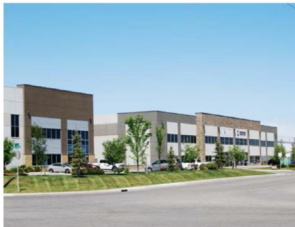
Photos: Examples of Industrial General
