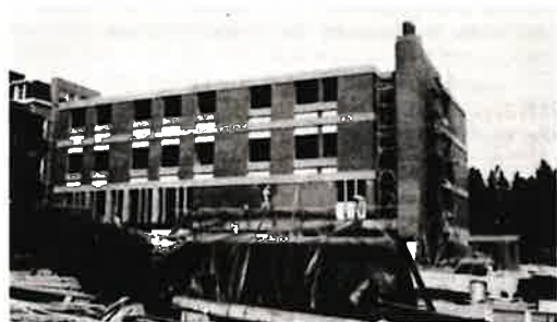
South wing under construction, 1966.
