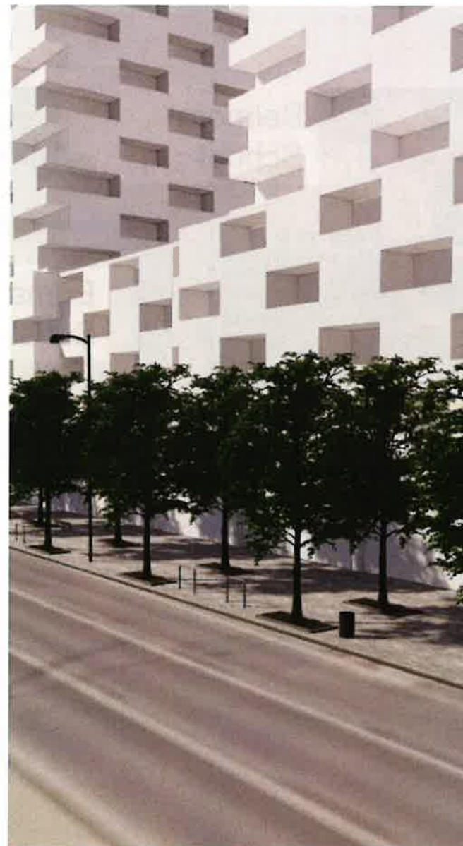
Fig 15. Enhanced public realm along 16th Avenue makes commercial uses viable and enables community gathering.
