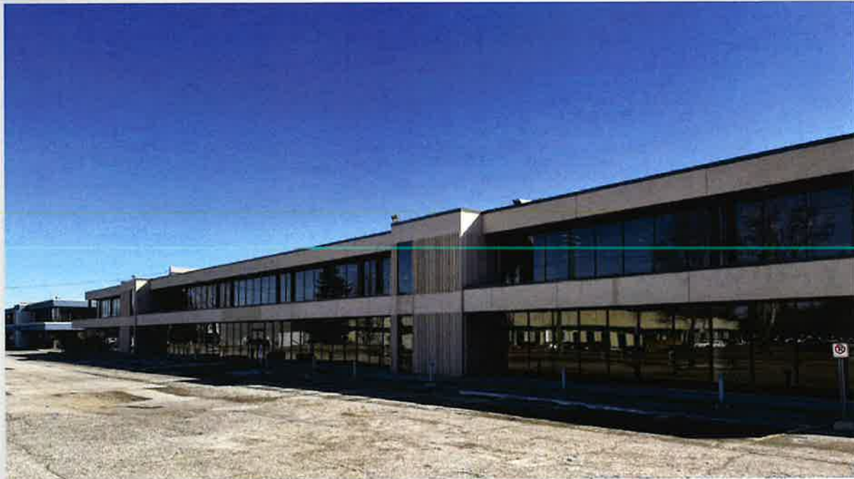
Front of Building
