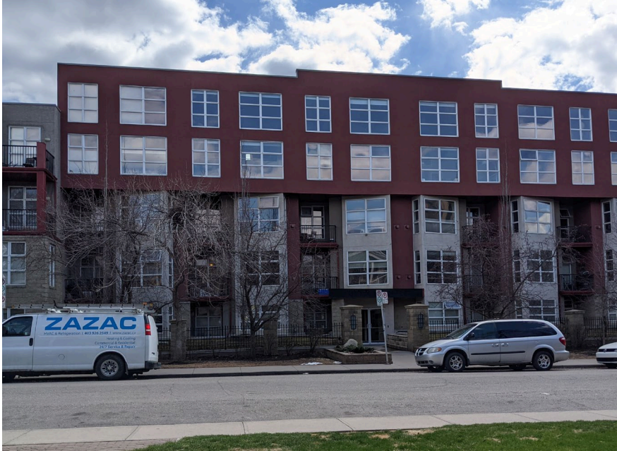
Photograph 3. XOLO (315 24 Avenue SW), a condominium project located directly adjacent to the north of the subject parcel. This building is a 5-storey walk-up, conforming to the allowable density (3.5 FAR).
