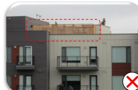
Screening should blend into the building design, rather than draw pedestrians' attention to the screen.
