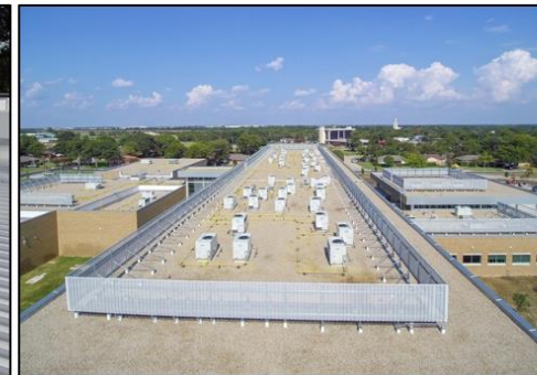
Screening a large area of rooftop equipment with metal rooftop screens.
