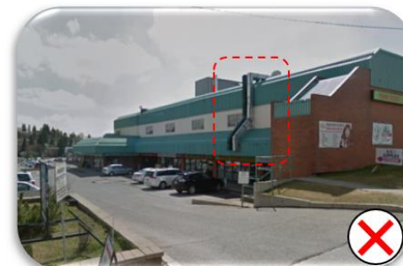
Equipment should be located out of view of public spaces, otherwise camouflaged or screened.
