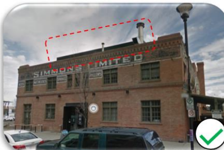
Equipment is partially screened, and partially exposed in a way that is harmonious with the building.
