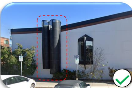
Wall mounted equipment is camouflaged with materials that enhance the building architecture.
