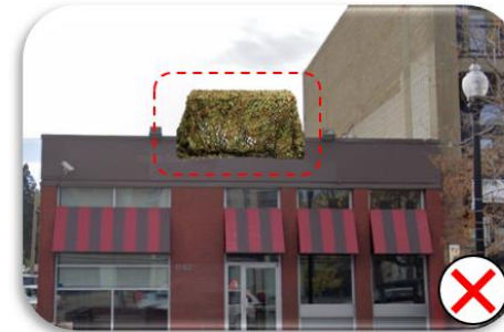
The attempted camouflage is not harmonious with the building and does not conceal the equipment.
