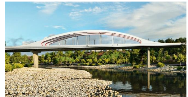
Tied arch (below deck structure)
