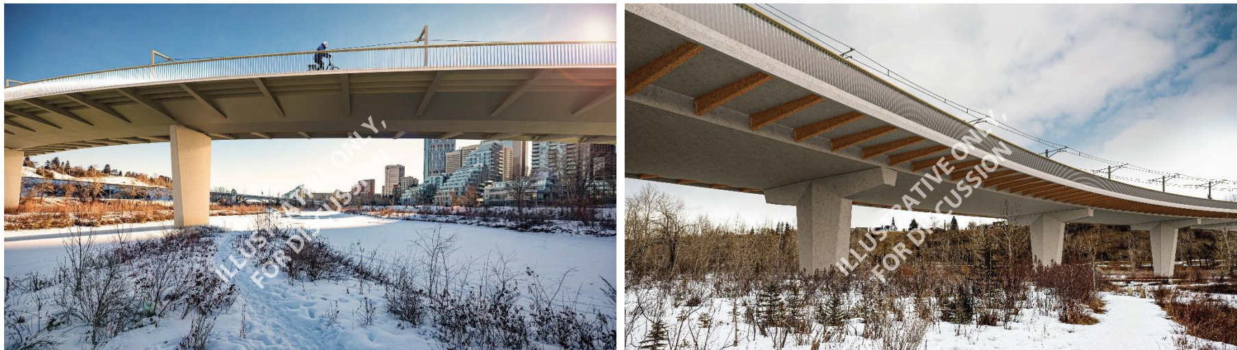
Conceptual renderings that illustrate what the bridge might look like with multi-use pathways on the outer deck. Pathway configuration allows for a thinner outer deck and open railings that make the bridge appear thinner and lower profile, hiding the inner structural beams.
