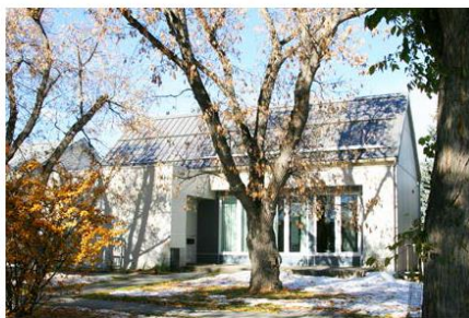
Photo: Mature trees provide shade, protection and visual interest on this residential site.
