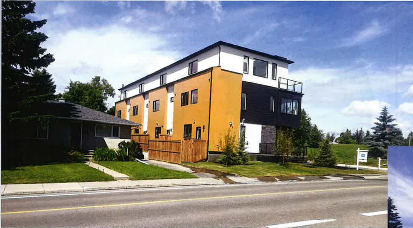
View of neighbouring M-CG development looking NORTHWEST from Spruce Drive
