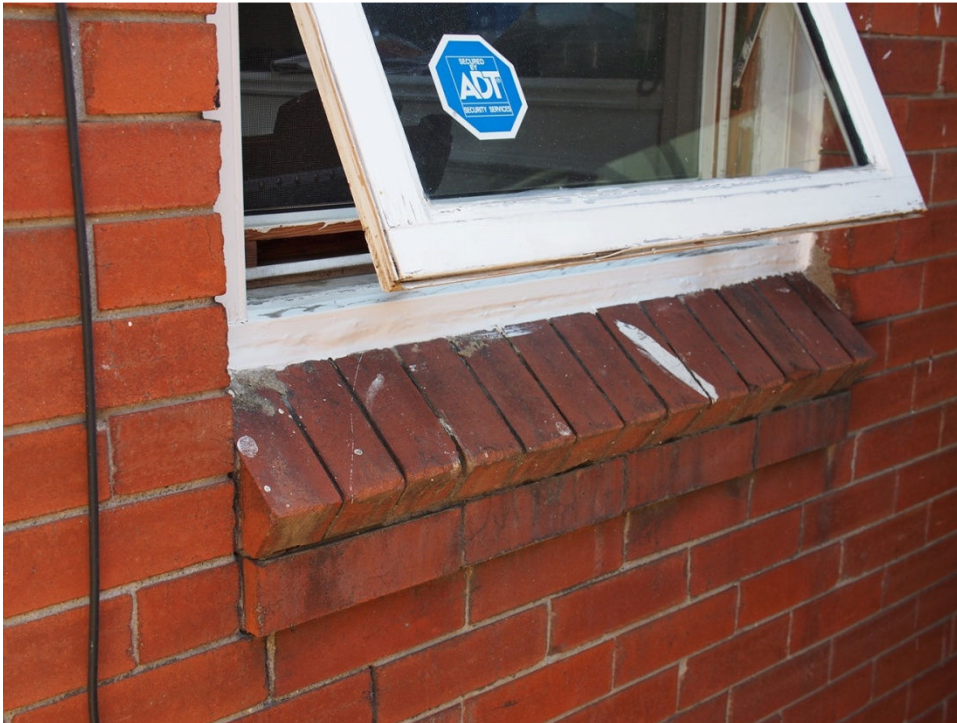
(Image #2.7 – Typical first-storey brick detail below window sill)
