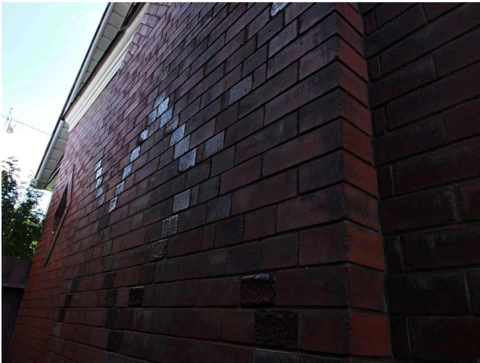
(Image #2.13 – Exterior of chimney, showing “XX” header pattern in alternate brick)
