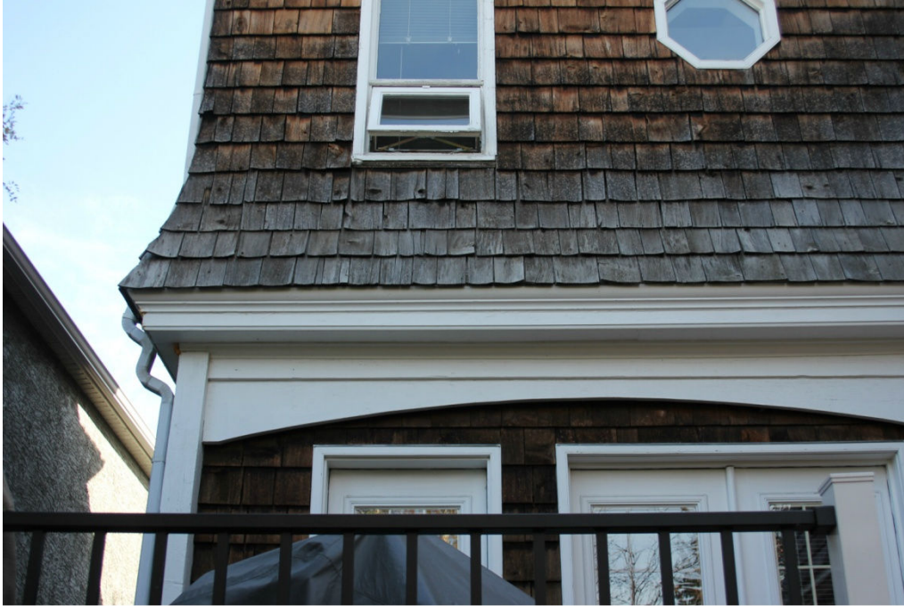
(Image #2.14 –Flared second storey wall on west façade; wood cornice; posts and decorative arch from original porch)
