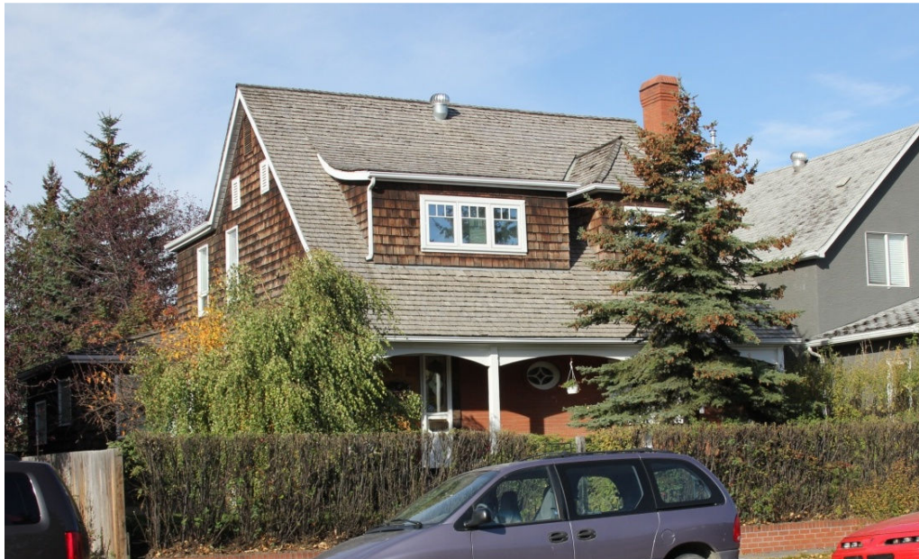
(Image #2.3 – South and east façades, showing roofline alteration to accommodate second storey addition)
