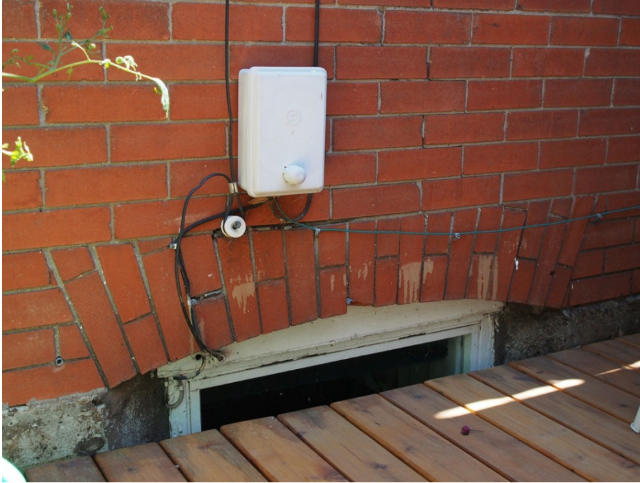
(Image #2.8– Typical basement window arch)
