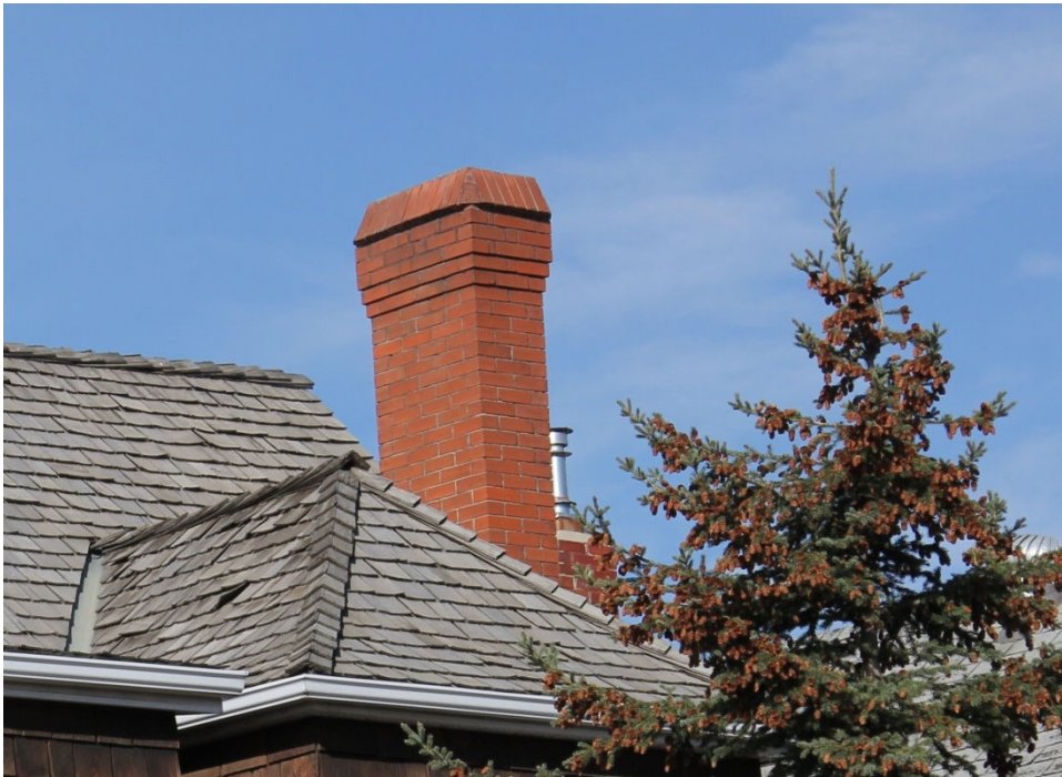
(Image #2.11 – Corbelled brick chimney with angled cornice)
