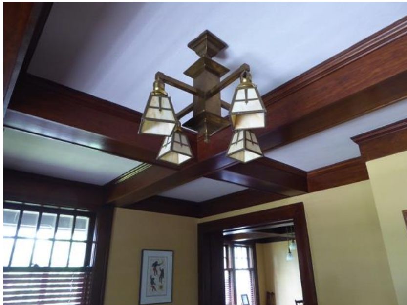
(Image 7.6 Example of extant original Douglas Fir crown moulding and ceiling beams in living and dining rooms)
