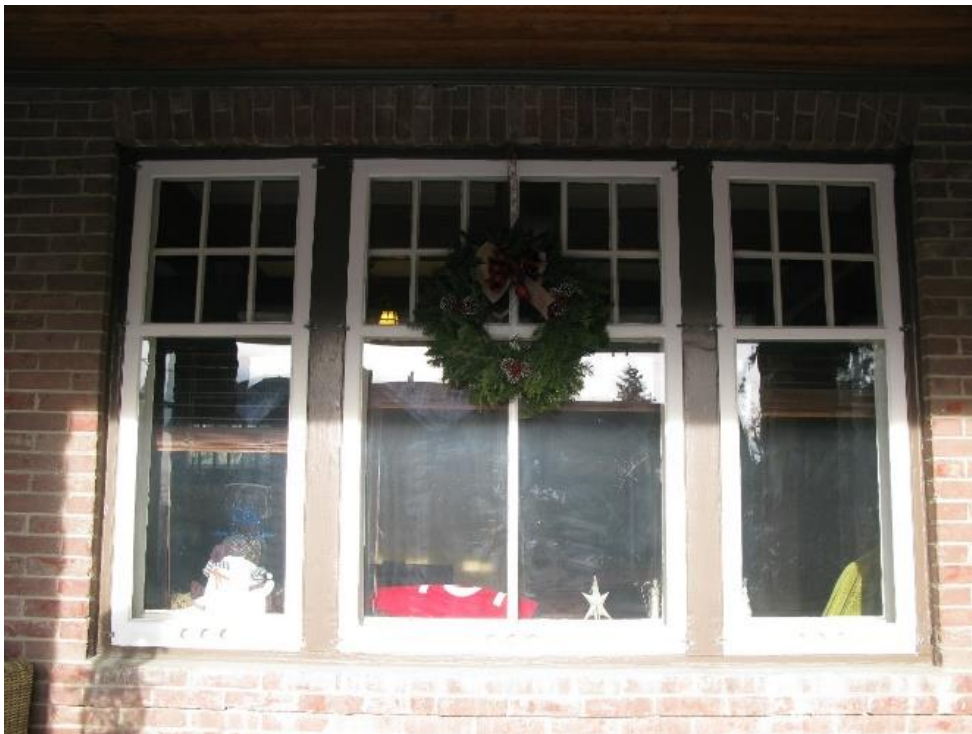
(Image 1.5: triple assembly consisting of a 12-over-1 flanked by 6-over-1 wood windows with sill and flat gauge lintel in concrete brick)
