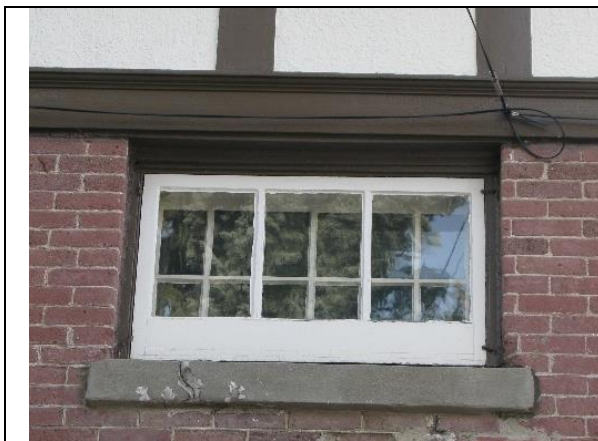
(Image 4.3: 12-pane wood window with concrete sill)
