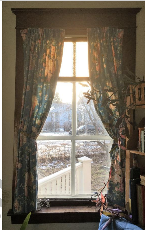
Image 3.2: Example of original wood window casing
