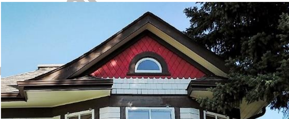
(Image 2.2: Detail of front lower cross gables with moulded eaves with return; half-moon architectural window, wood shingle and diamond-patterned shingle cladding; plain frieze)
