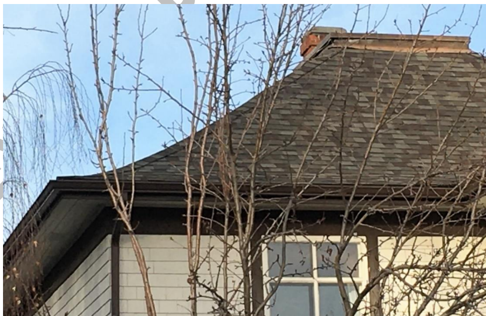
(Image 2.4: Detail of hipped roof with bell-cast (curved) eaves (at roof corners))
