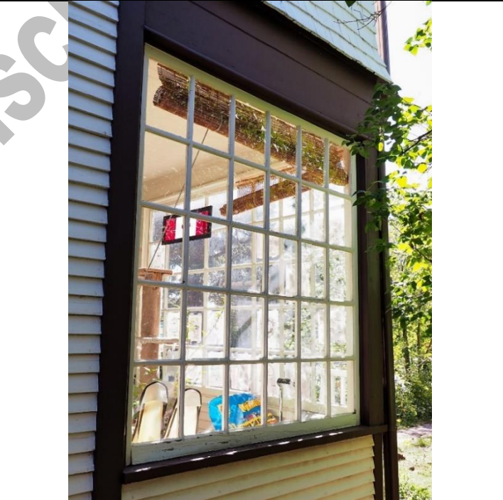
Image 2.14: Example of fixed, multi-light wood sash windows on inset veranda
