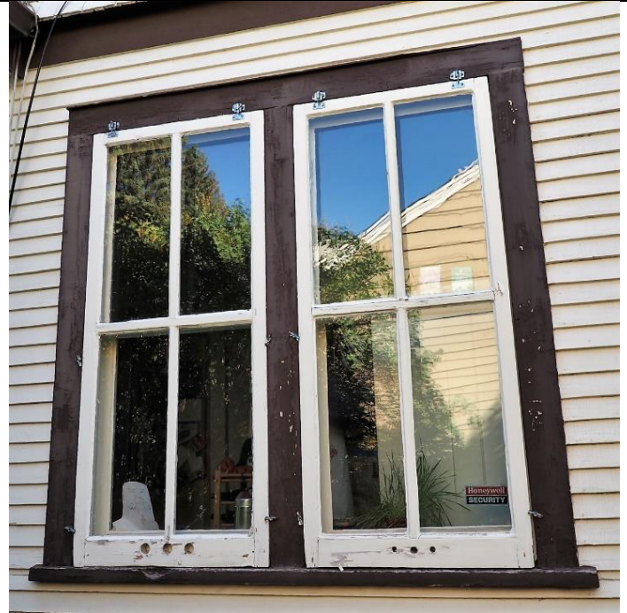
Image 2.12: Example of two 1-over-1 single hung wood sash windows in a double assembly format and 4-light wood storm windows
