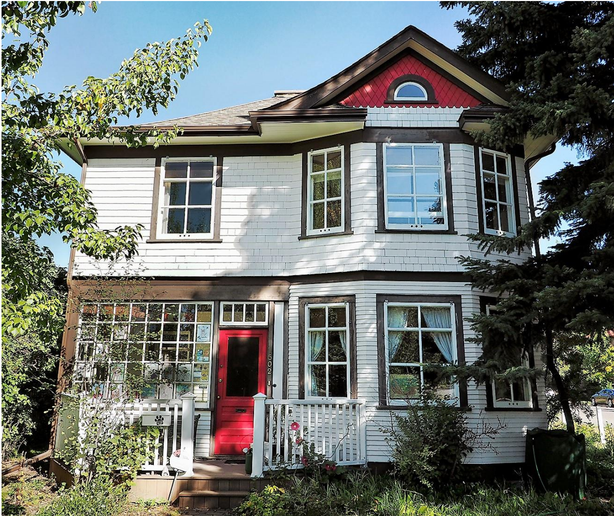
(Image 2.1: Front (south) façade)
