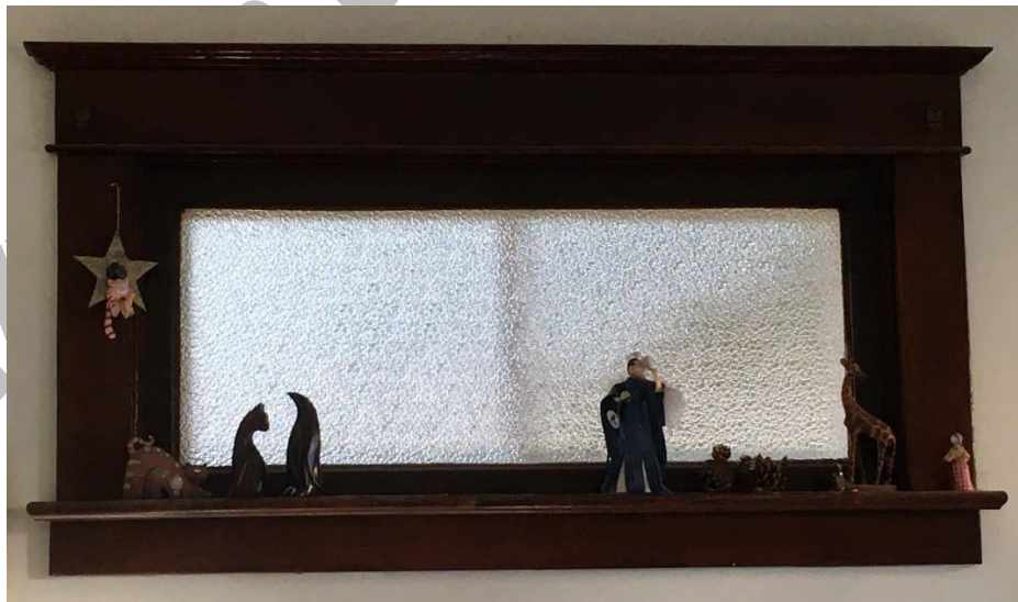
(Image 3.3: Example of original wood window casing)
