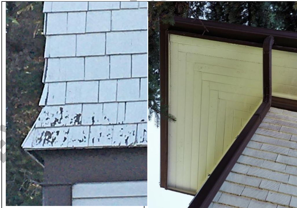
Image 2.6: Detail of flared wood shingled corner on second storey
