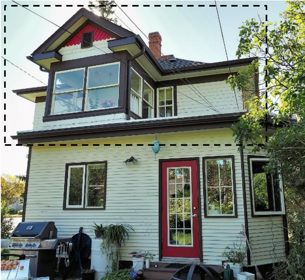
(Image 2.10: Rear (north) façade showing cross gable with wood shingle and shingle diamond-pattern; enclosed balcony with two of three double assemblies of 1-over-1 single hung windows and 1-over-one single hung window. Note: Regulated portions are in area with dashed border.)
