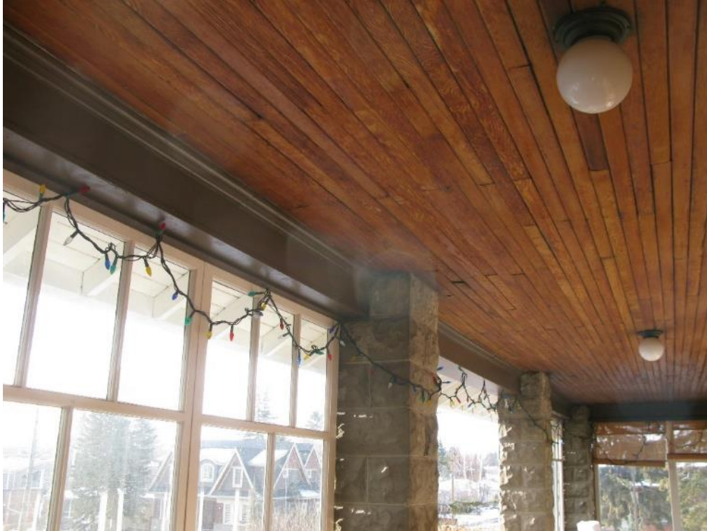
(Image 1.4 Enclosed portion of verandah: tongue-and-groove ceiling, hollow rock-faced concrete block clad support pillars, wood header)
