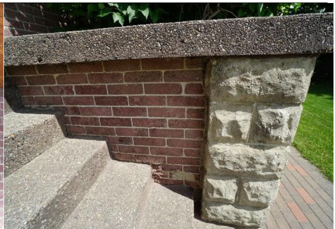
(Image 1.8: Detail showing exterior front stairs: walls of concrete bricks laid in stretcher bond and hollow rock-faced concrete blocks)
