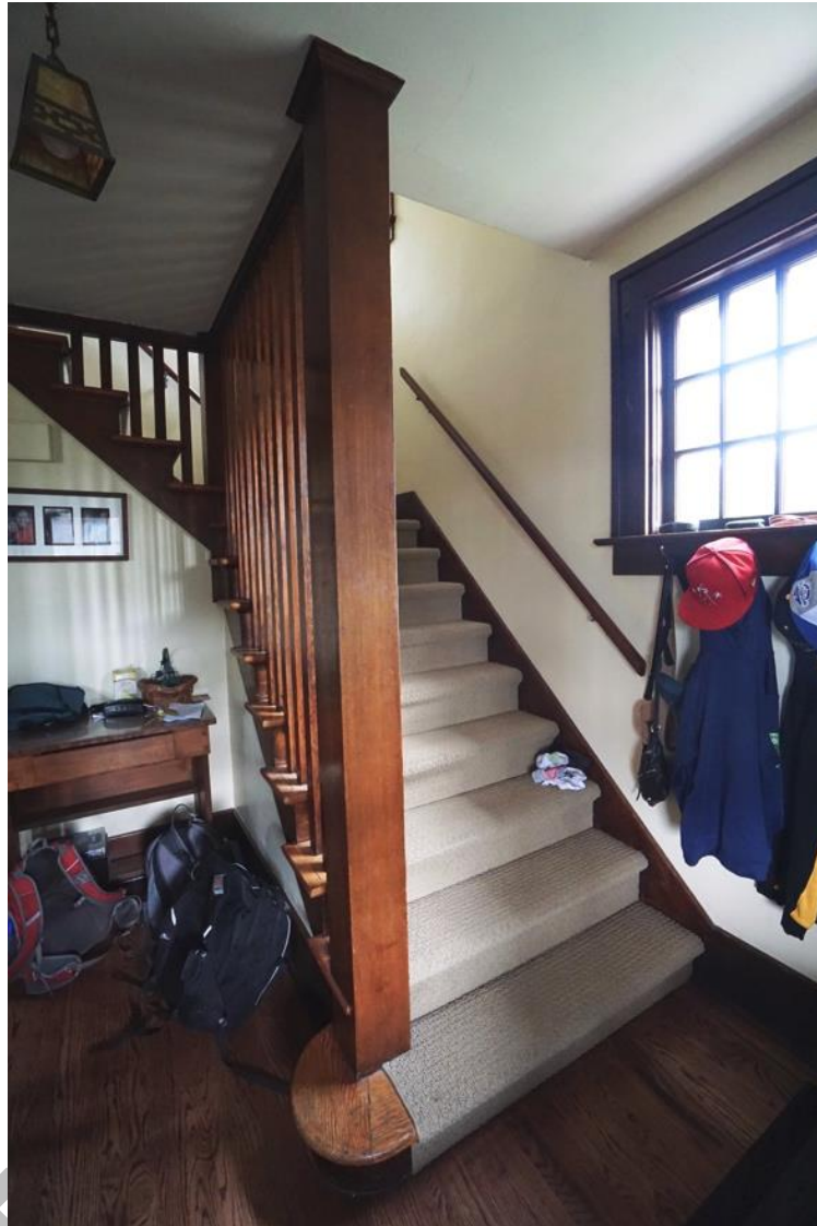
(Image 7.7: Quarter-turn closed staircase to second storey with Douglas fir stair rail, newel, and balustrade; example of a window casing)
