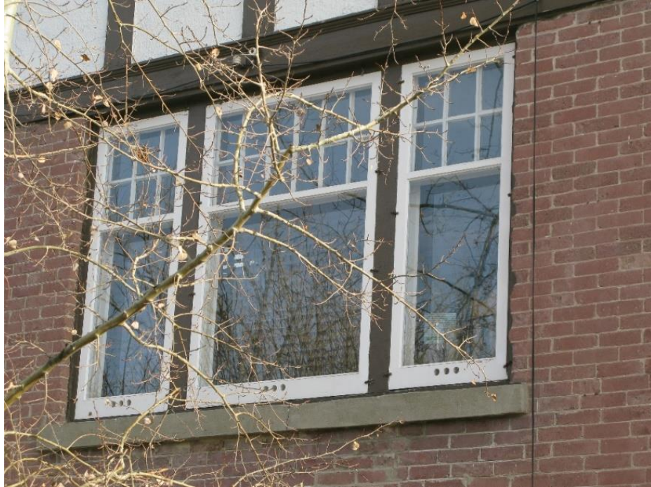
(Image 3.2: triple assembly consisting of a 12-over-1 flanked by 6-over-1 wood windows, with concrete sill; continuous wood band with decorative trim)
