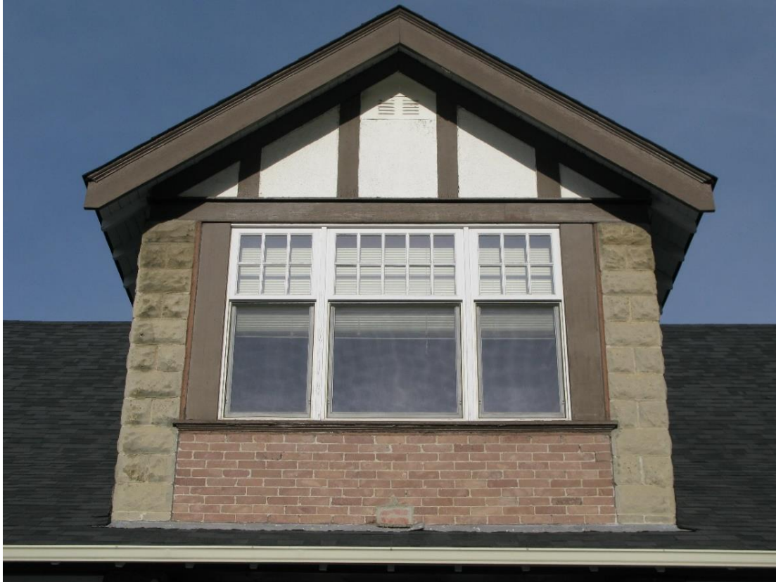
(Image 1.6: detail of second storey porch extension, stretcher bond concrete brick cladding with hollow rock-faced concrete block corner columns; stucco and wood mock half-timbering)
