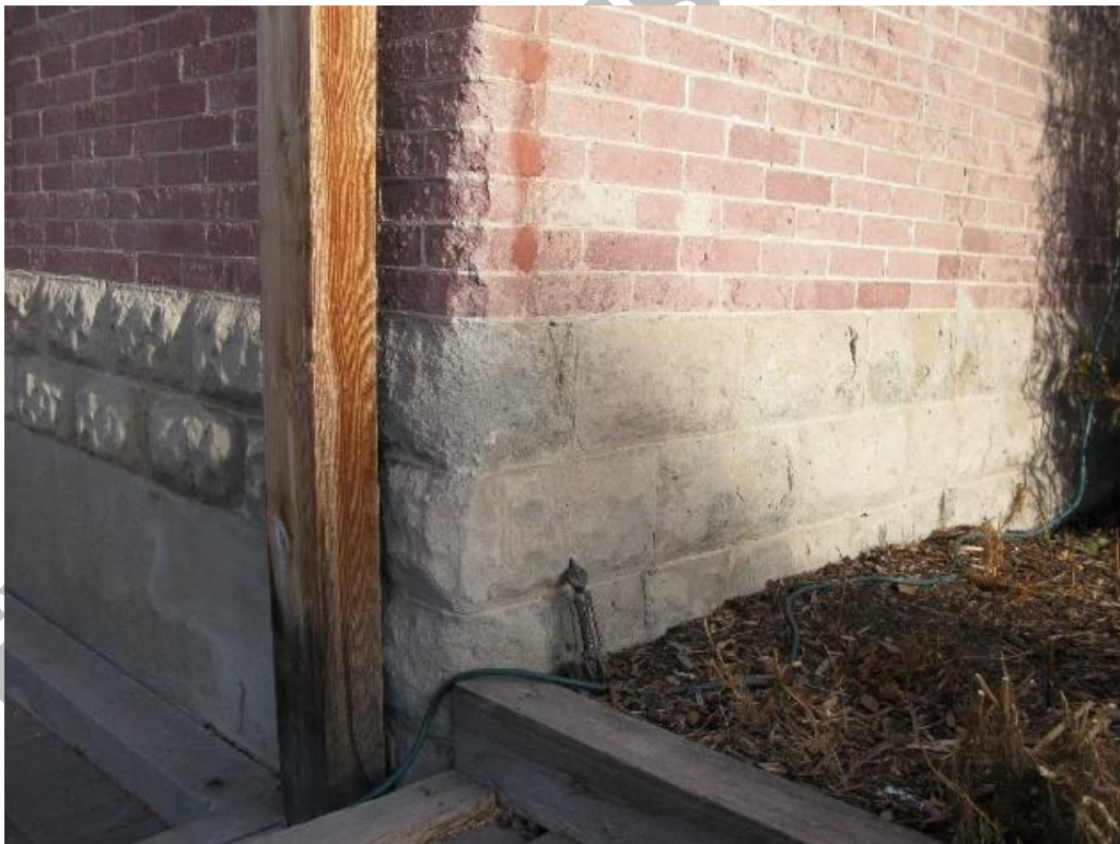
(Image 1.3 Stretcher bond concrete brick cladding; continuous hollow rock-faced concrete block band (three rows in south-facing façade, transitioning to two rows))
