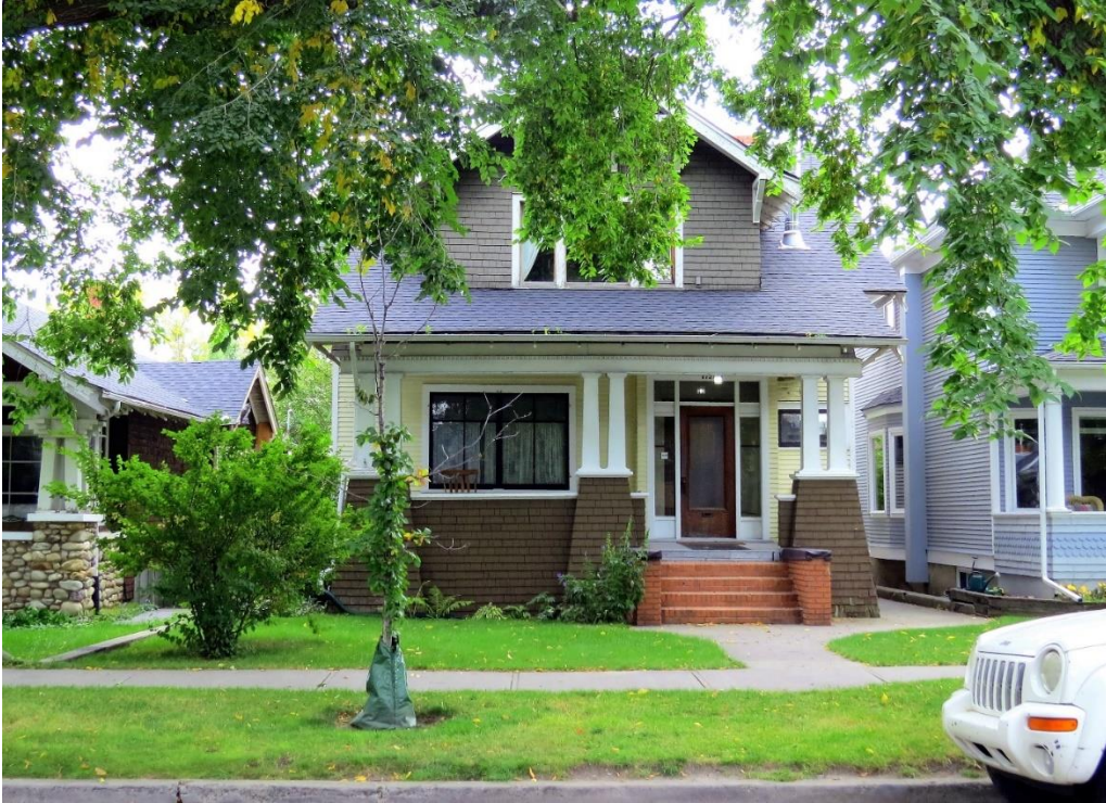
(Image 2.1: North (front) façade showing front cross-gable dormer and full-width front veranda)
