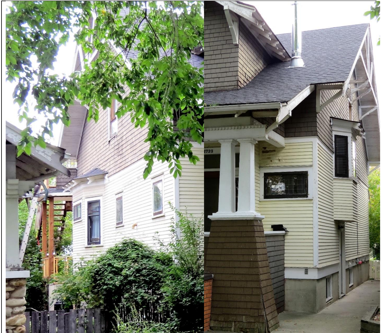
Image 2.5: Hip-roofed bump out on east façade, bevelled wood and shingle cladding, exposed rafter tail; and example of 1-over-1 single hung profile and 2-light fixed profile
