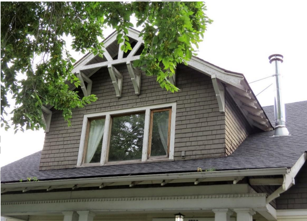
(Image 2.2: Detail of front cross-gable dormer on high-pitched, side gable roof; stick work (gable peak); overhanging eaves with exposed rafter tails, wood brackets, wood tongue-and-groove soffits and moulded frieze; projecting verges with vergeboards with decorative ends)
