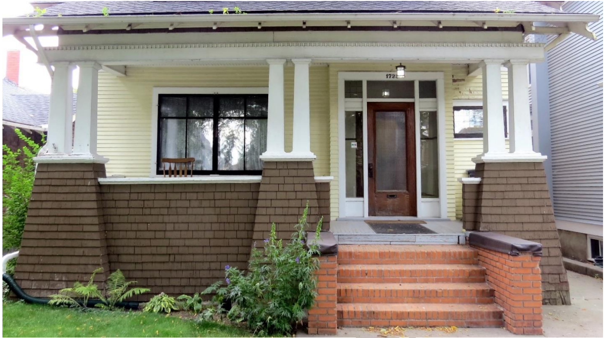
(Image 2.3: Detail of full-width shingle clad, front veranda with closed balustrade, tapered piers and twinned, tapered posts supporting moulded entablatures)
