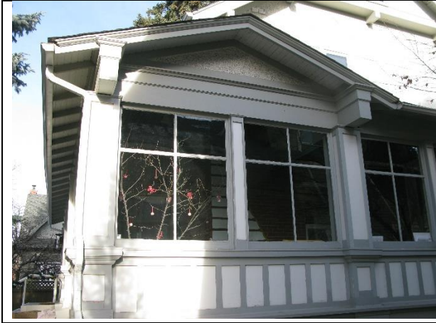
(Image 2.7: Side-gable roof with outriggers and moulded capitals (veranda))
