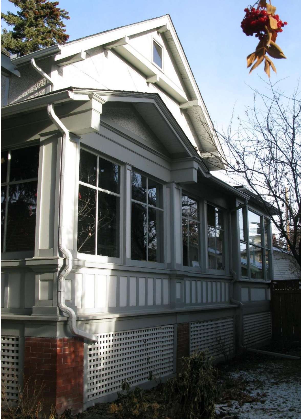
(Image 2.2: Oblique view of south facade)
