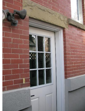
(Image 2.12: Example of door opening with sandstone lintel)
