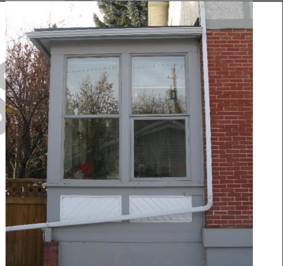
(Image 2.10: north side of the rear porch extension)
