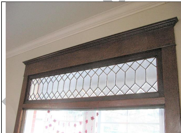
(Image 3.4: Front window topped by leaded glass in geometric pattern. Example of window casing)
