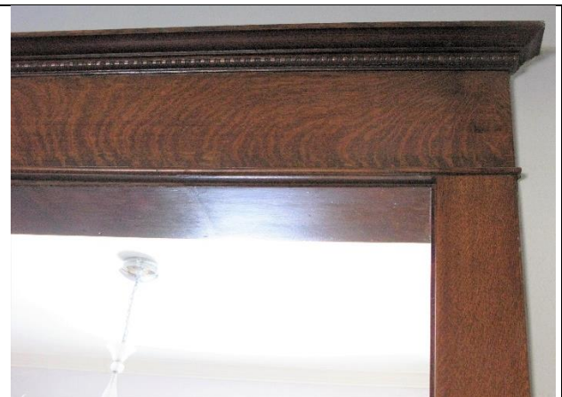
(Image 3.5: Detailing on a typical door trim and casing)
