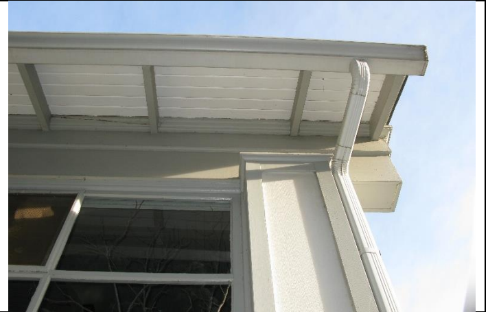
(Image 2.8 Verandah eaves, wood tongue-and-groove soffits, exposed rafters)
