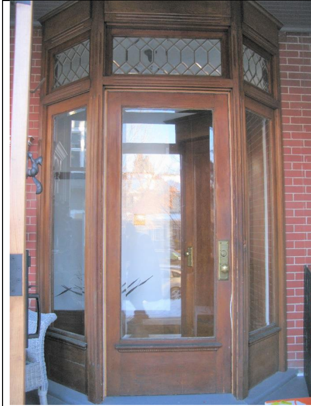
(Image 3.2: three-sided front vestibule comprising moulded oak frame, oak front door and two oak side walls filled with beveled glass, transoms across all three sections of leaded glass in geometric pattern)
