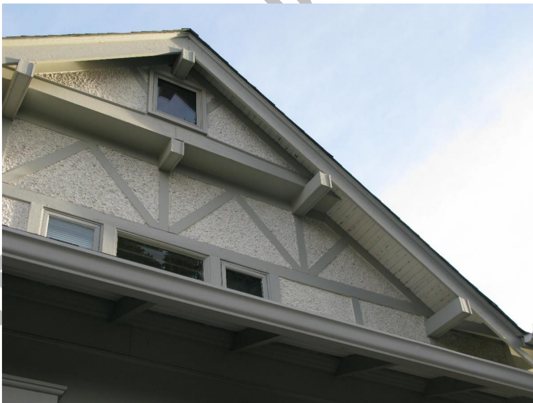
(Image 2.6: Front-facing portion of cross-gable roof, wood tongue-and-groove soffits, exposed rafters, wood mock half-timbering)
