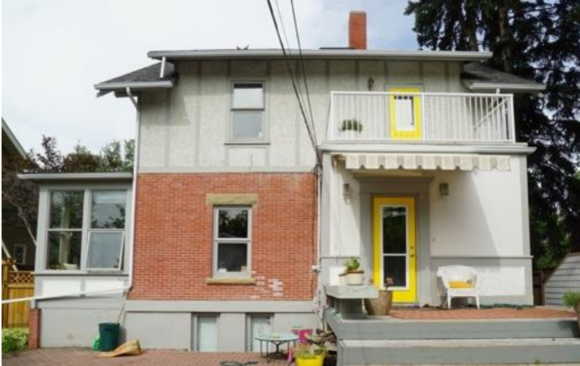
(Image 2.5: East facade)
