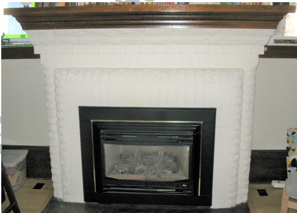
(Image 3.8: brick and stucco (living room) fireplace, with crenellated and corbelled top, molded oak mantelshelf)
