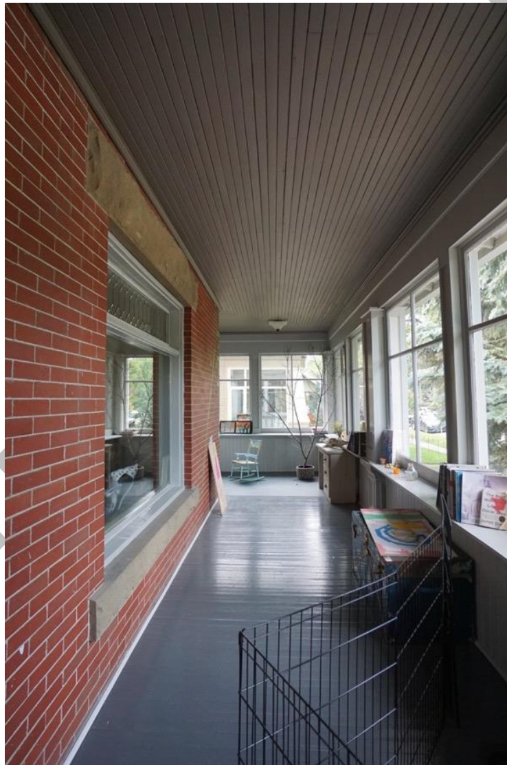
(Image 3.1: Veranda, showing plank flooring and tongue-and-groove ceiling; front window, topped by leaded glass in geometric pattern, with sandstone lintels and sills)
